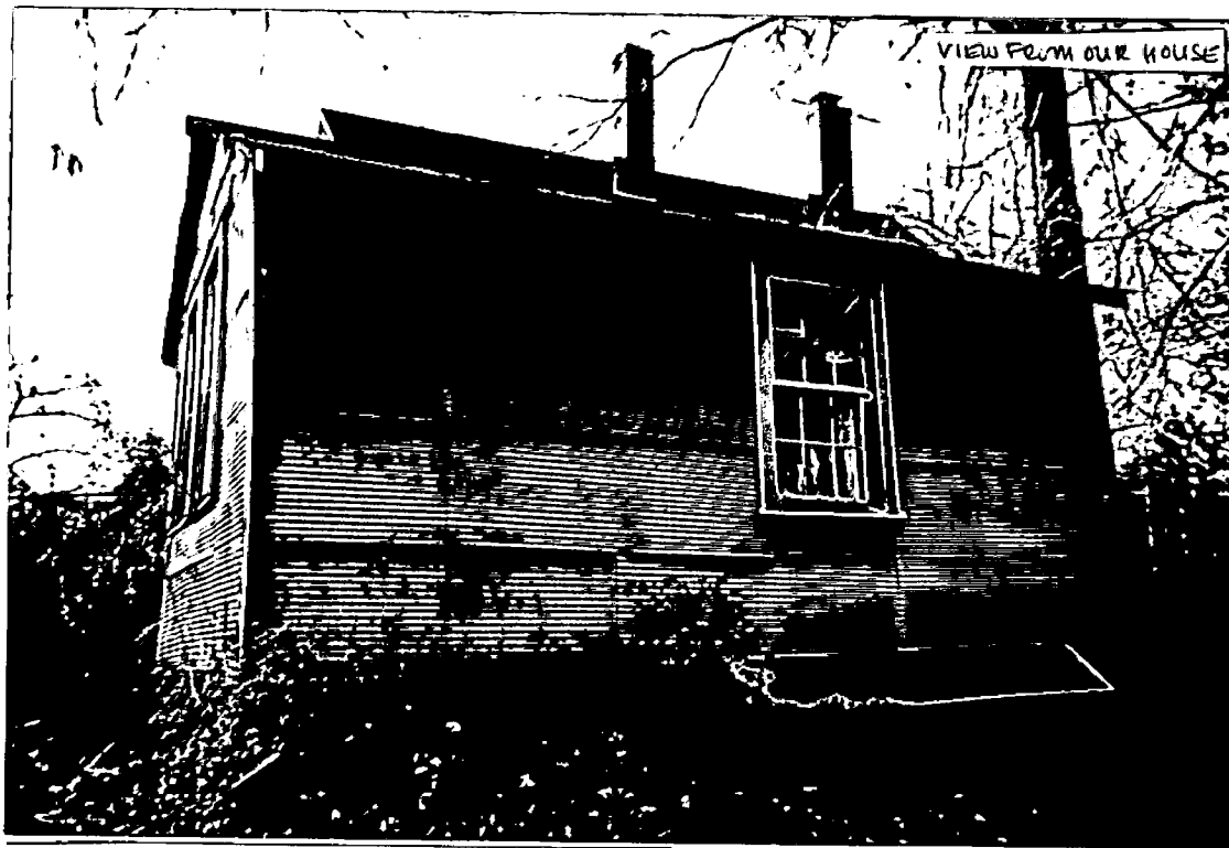
Detail: SIDE OF GARAGE FACING OUR PROPERTY
