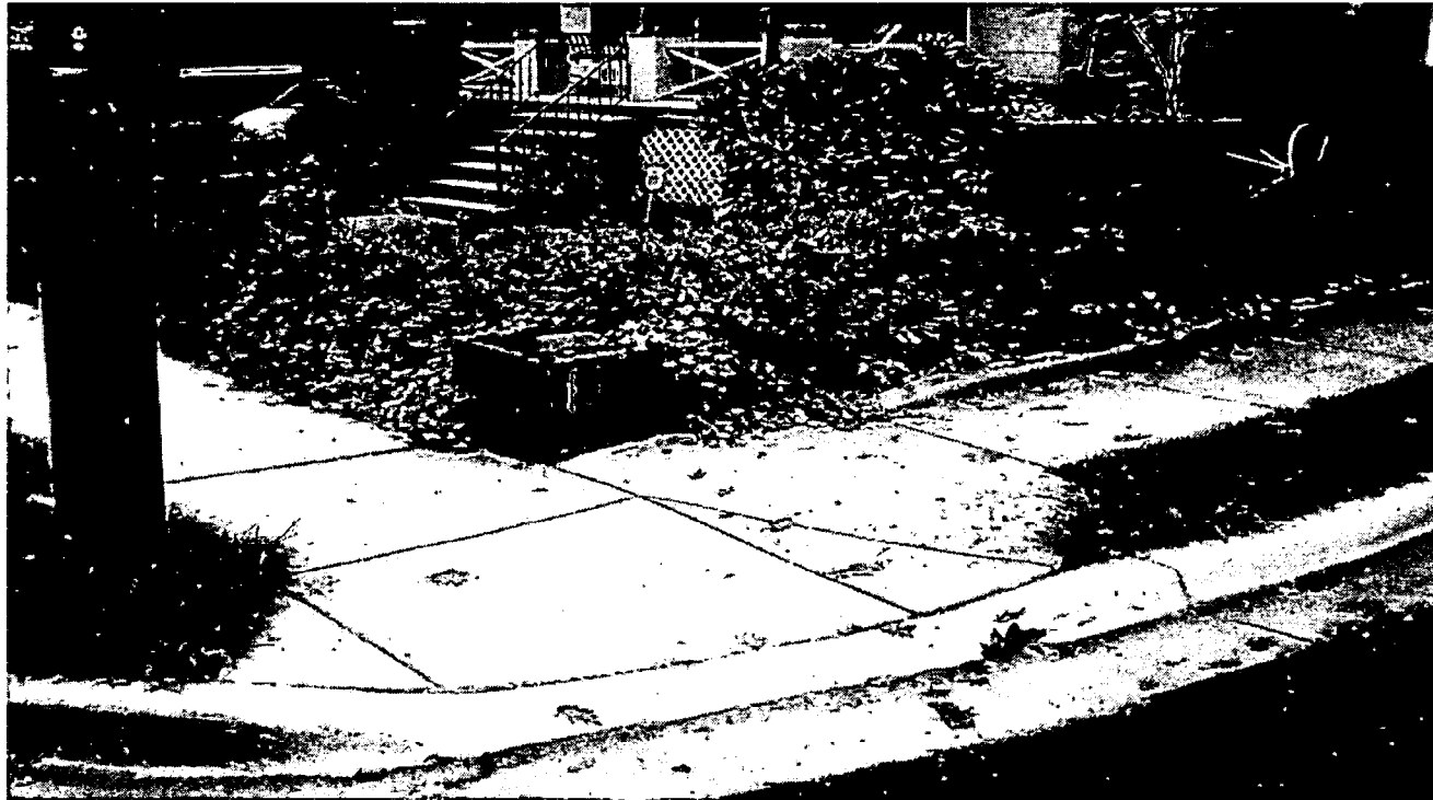
1411 Maple Ave at the corner of Maple and Valley View. There is a low wall along Valley View. There is no wall along Maple.
