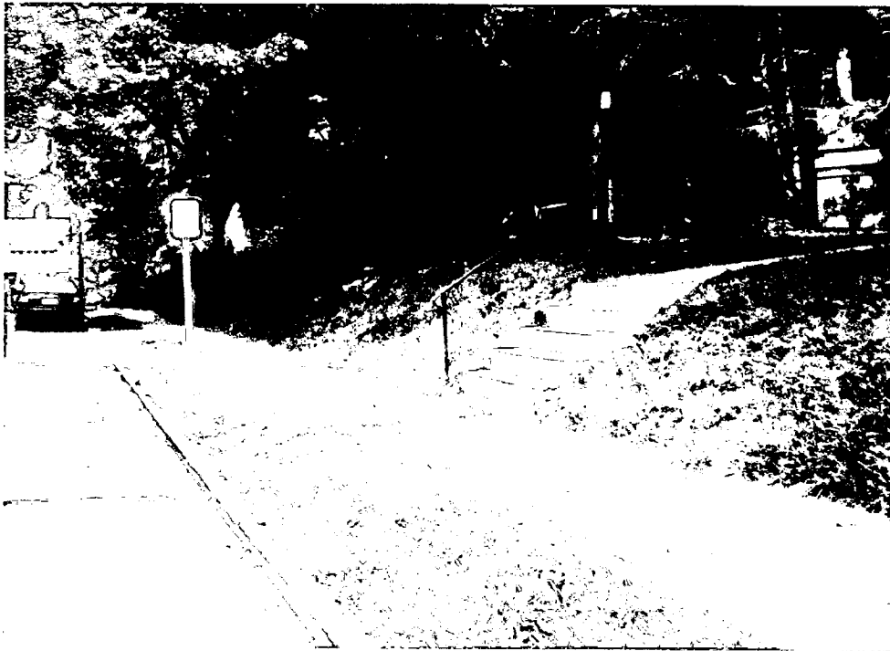
A view from the stairs along the side walk. The wall will start on the left of the stairs.
