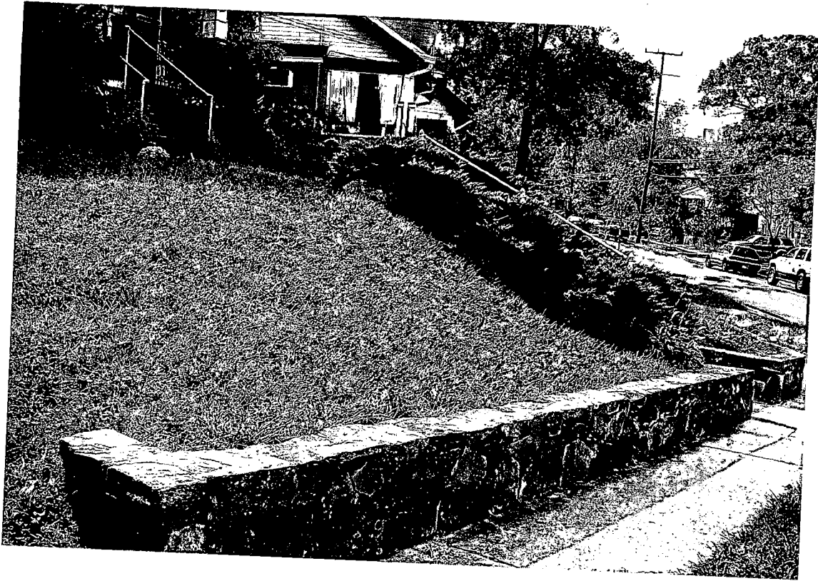
Retaining Wall - 219 Park Avenue, Takoma Park H.D. Adjacent to 25 Holt Place.
