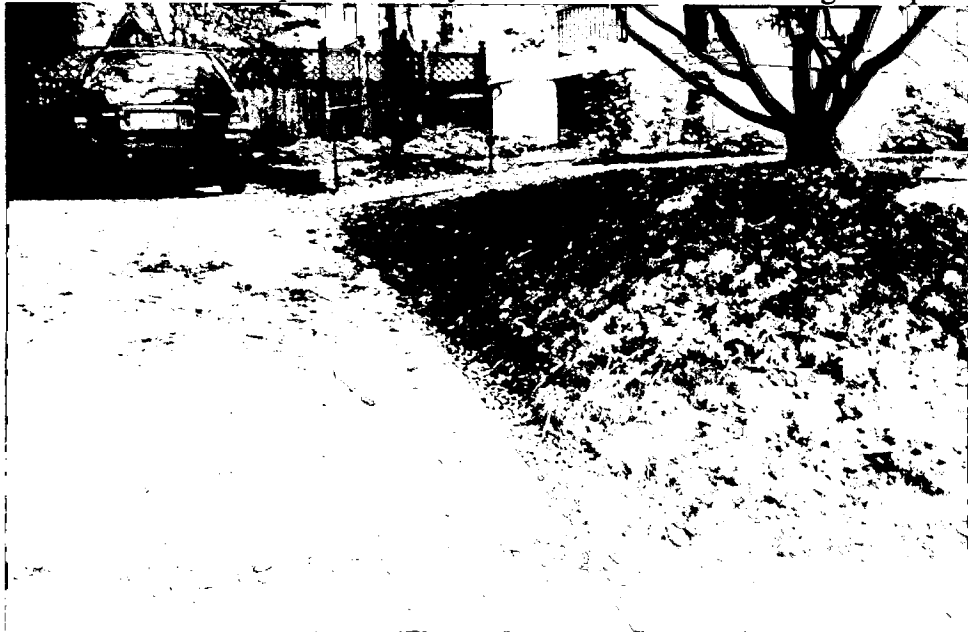
A view from the sidewalk up the driveway. The wall will end at the flagstone path.
