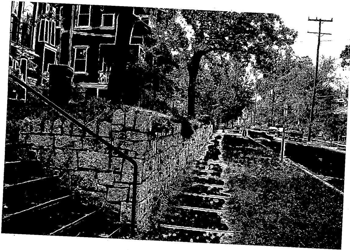
Retaining Wall, 217 Park Avenue - Takoma Park H. D. Adjacent to 25 Holt Place.
