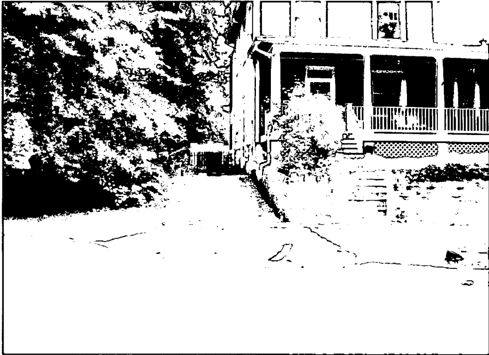
239 Park Ave at the corner of Park and Crescent. There is a wall to the right of the driveway and none to the left.
