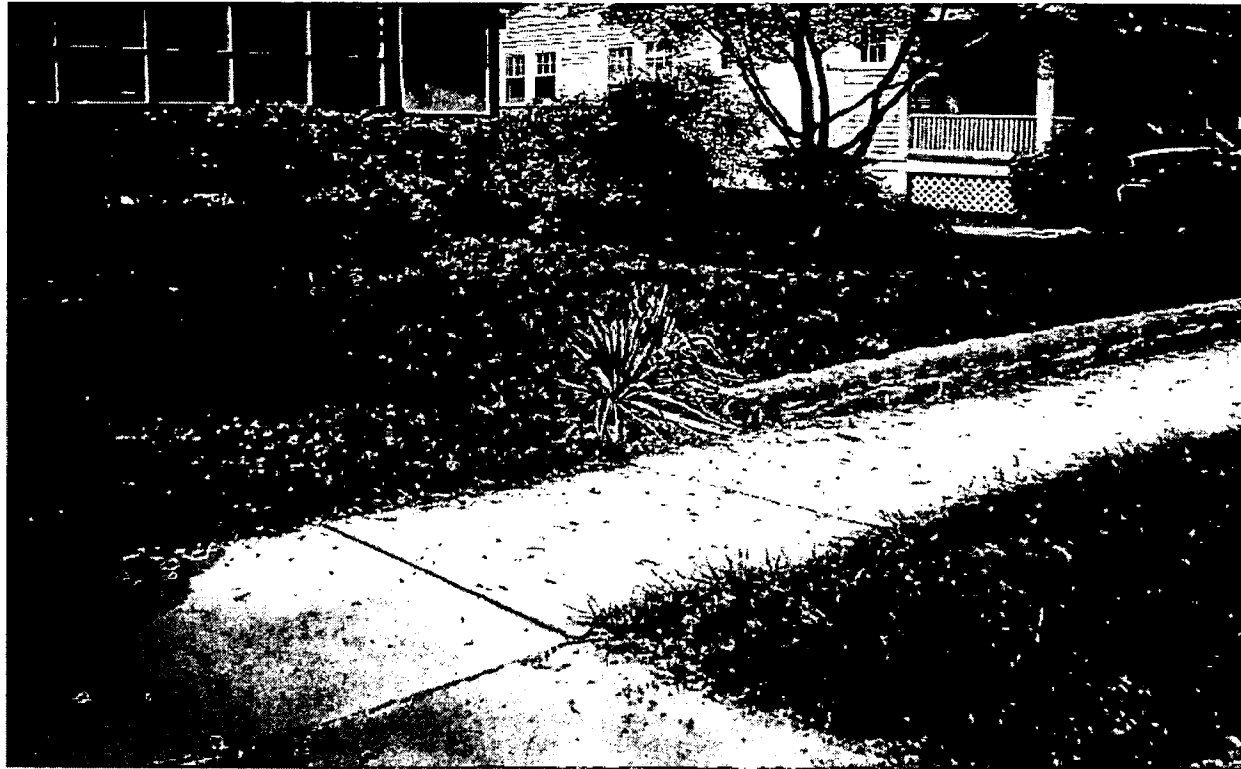
7316 Willow Ave. The wall stops in the middle of the front yard.
