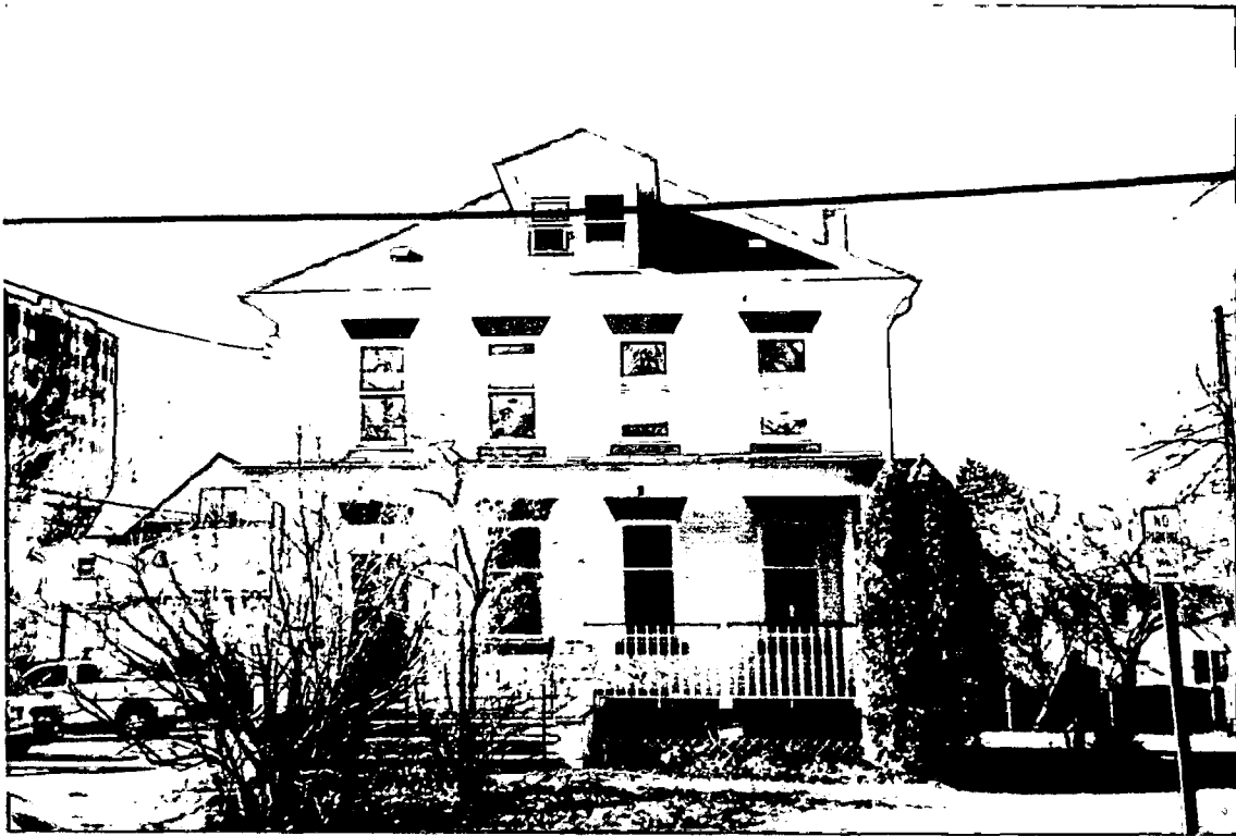
Photo No.1 The front elevation does not presently have an entrance sidewalk. It is proposed to replace the existing bushes in order to place a 4 foot wide sidewalk from the sidewalk at the street to the main entrance of the house as shown on the site plan (drawing page 2 of this application).
