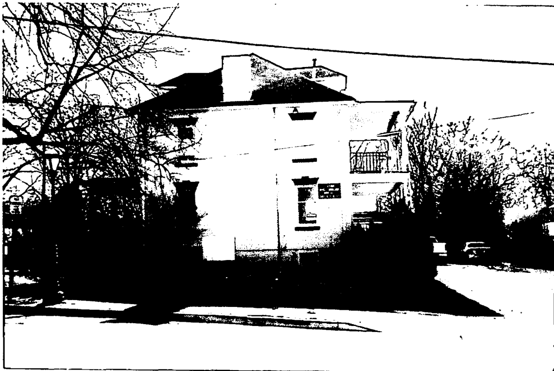
Photo No.2 The right side of the house as seen from Columbia Avenue remains unchanged except for the stairs in side the existing rear porch. The proposed rear porch stair would require the removal to the Juniper bush at the rear.
