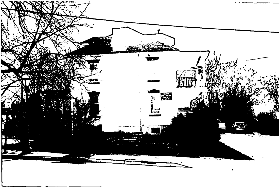
Photo No.2 The right side of the house as seen from Columbia Avenue remains unchanged except for the stairs in side the existing rear porch. The proposed rear porch stair would require the removal to the Juniper bush at the rear.
