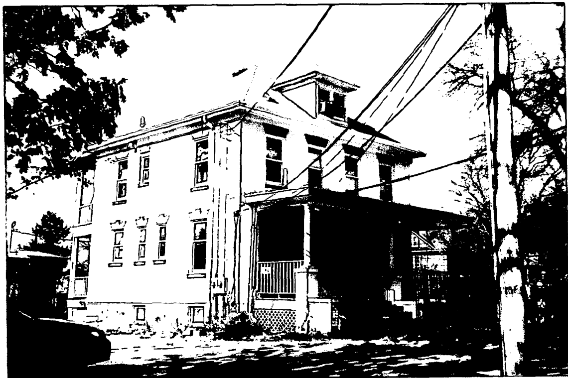
Photo No.4 The left side of the house at the parking area would remain unchanged except for the proposed pavers for the parking area.
