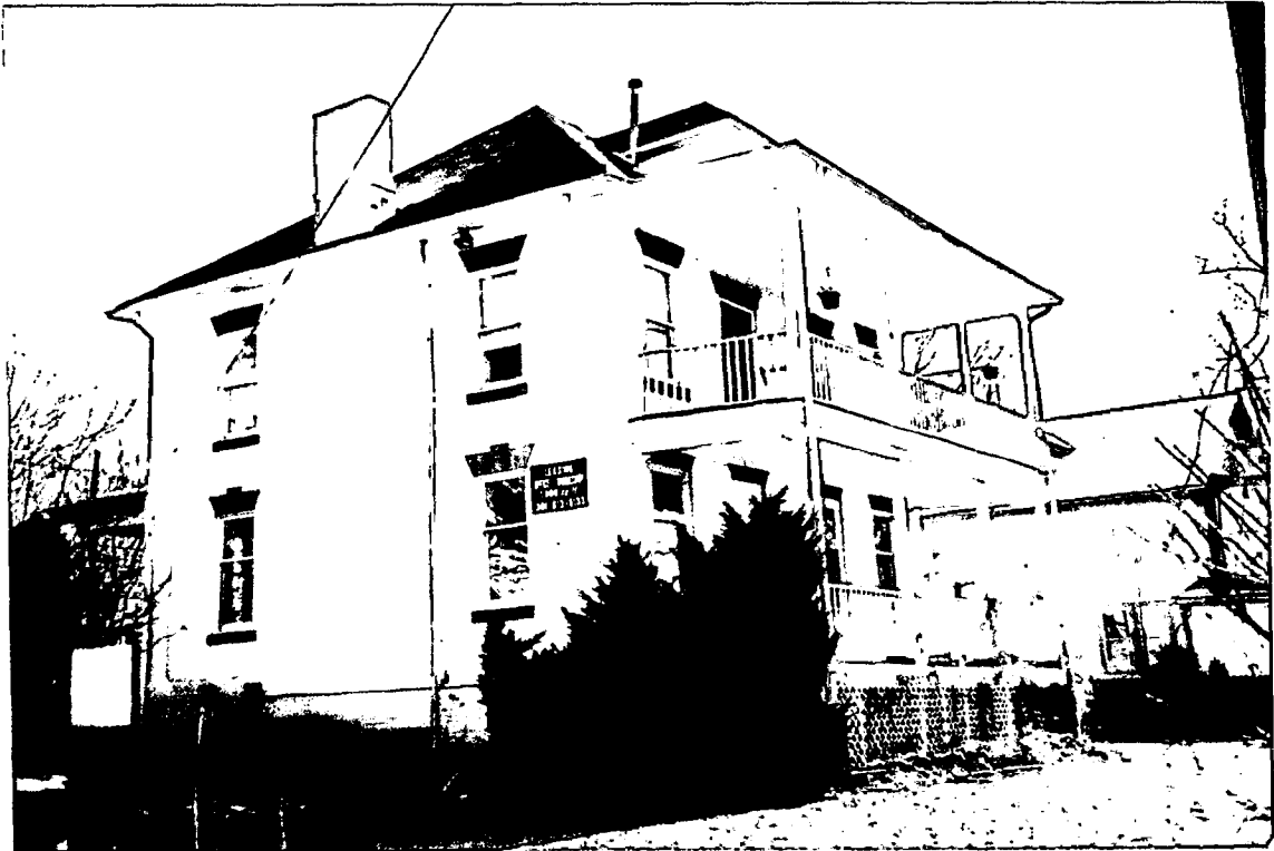
Photo No.3 It is impossible to get a direct picture of the rear of the house due to the limited space at the rear of the house. The only change to take place would be the addition of stairs inside the rear porch area that would run from the ground to the first floor porch and then from the first floor porch to the second floor porch.
