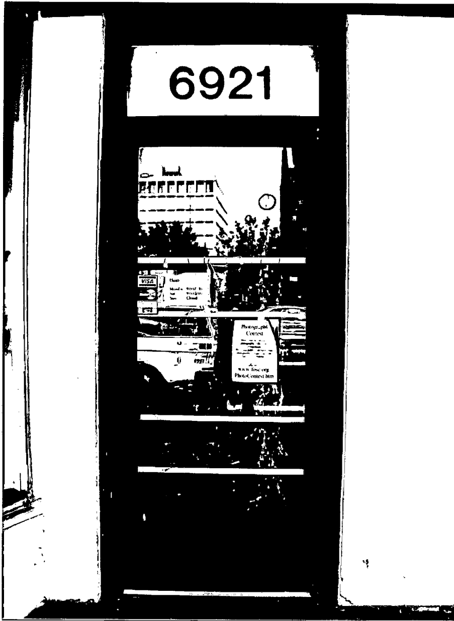
Picture 5 Adjacent Front Door
