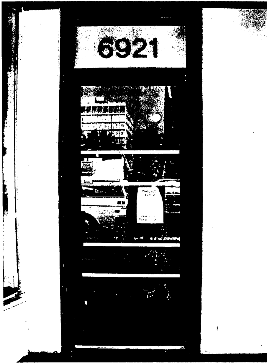
Picture 5 Adjacent Front Door
