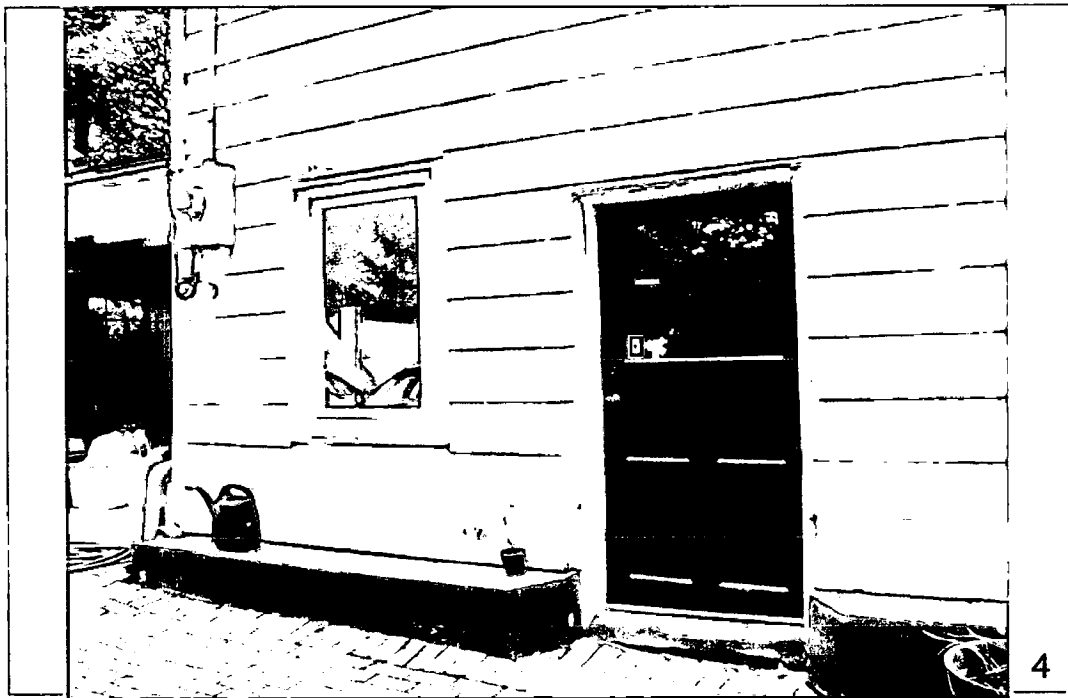
Detail: Concrete 'Ledges' along North side of Existing house
