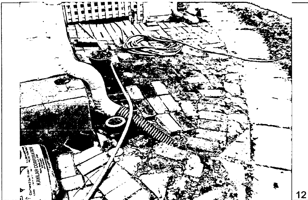
Detail: View of brick paving and flagstone path to Northwest of house
