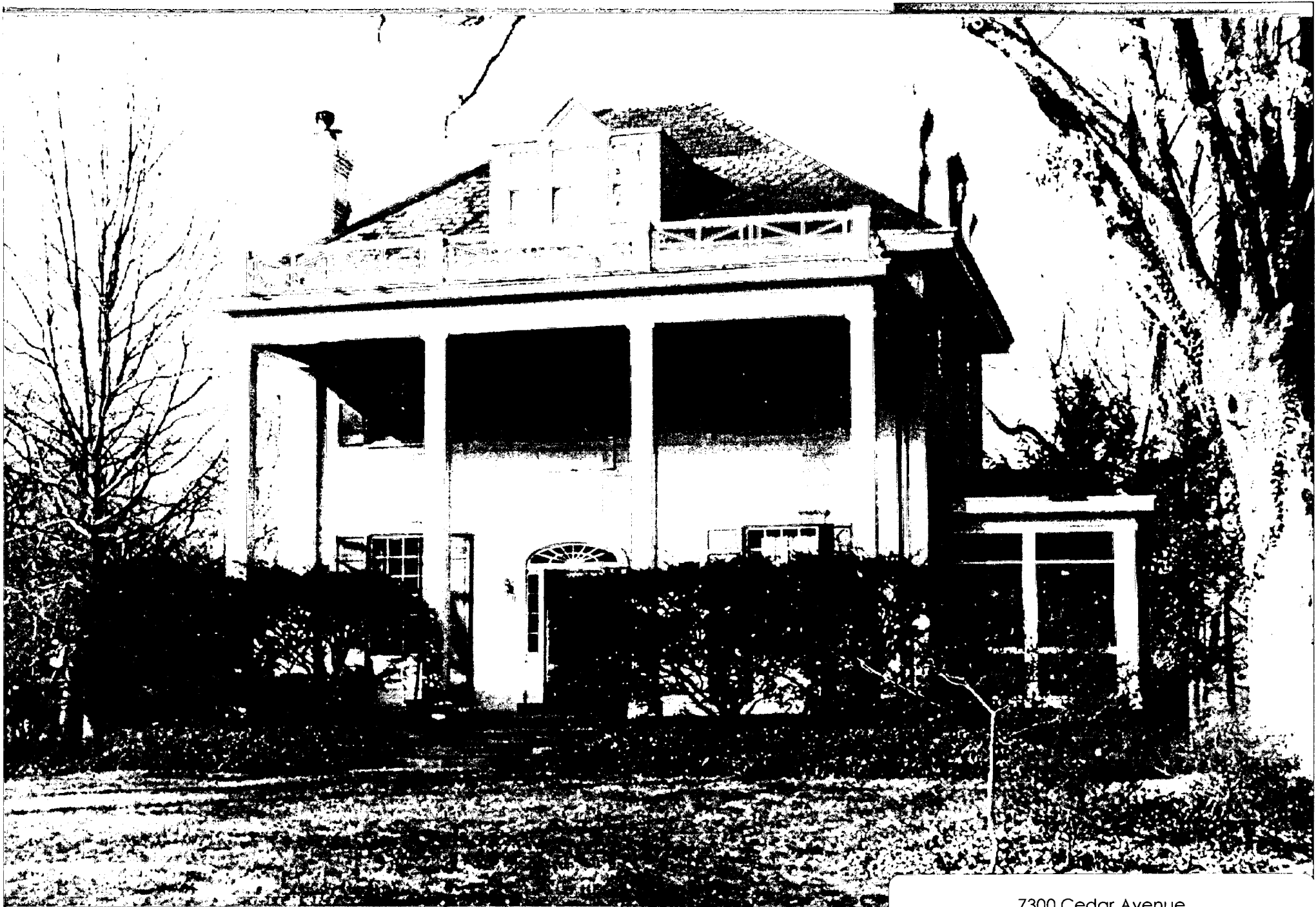
7300 Cedar Avenue South Façade w/1939 Porch Roof Railing
