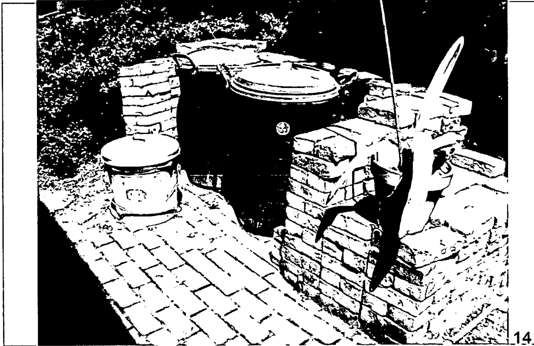
Detail: Brick 'surround' for garbage cans
