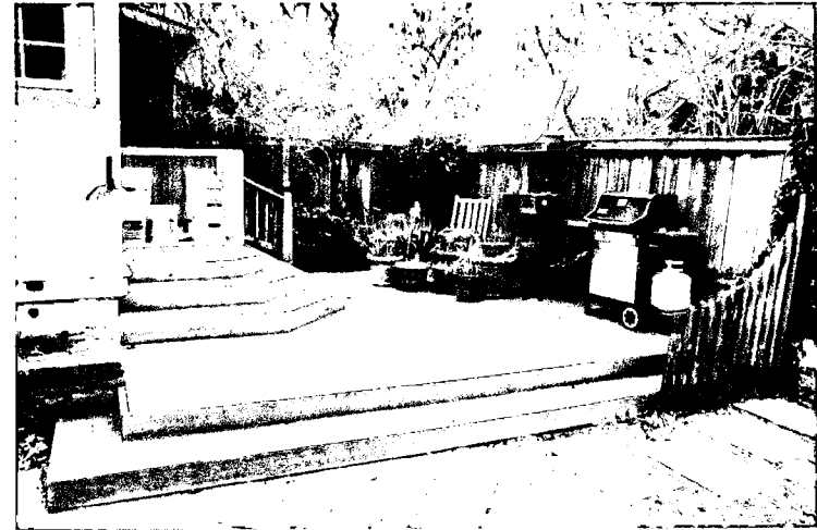
Deck to be removed
