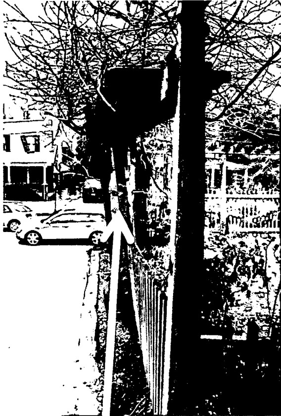
Structure no longer vertical
