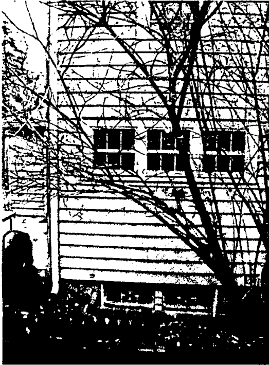
Side of house at driveway
