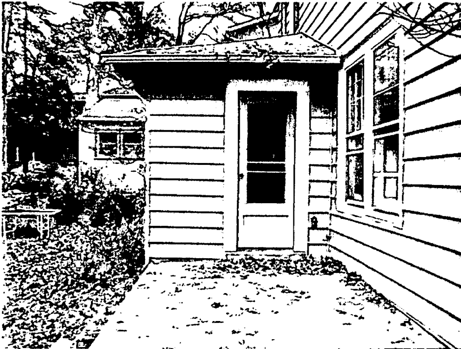
Existing concrete porch (future location of proposed screened porch, we would like to replace these windows with French doors in the future as connection from dining room to screened porch).
