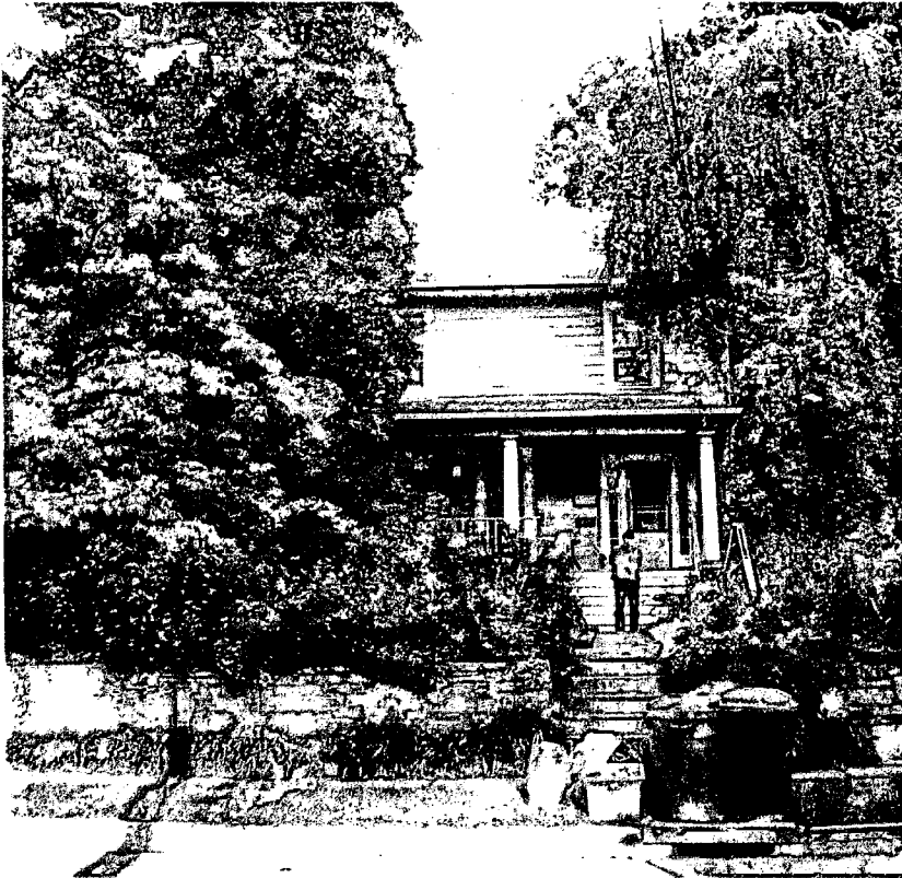
Front of home as viewed from Holly Ave.
