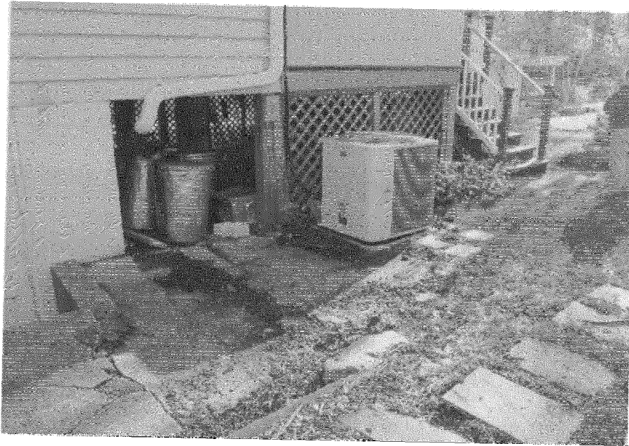
garbage area - add timbers to help with grading & drainage in this area
