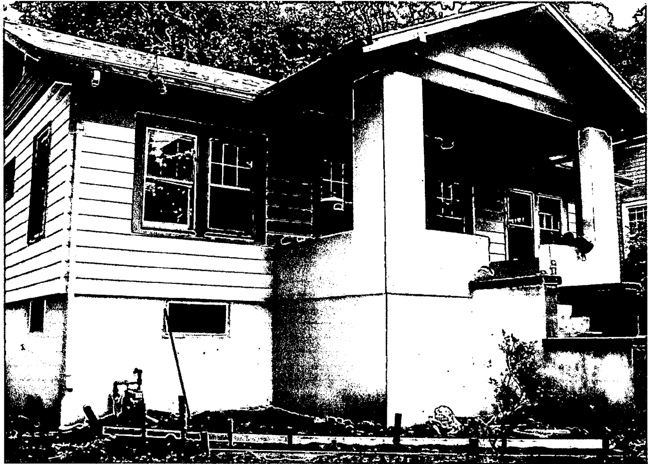
FRONT SIDE EXISTING VIEW
