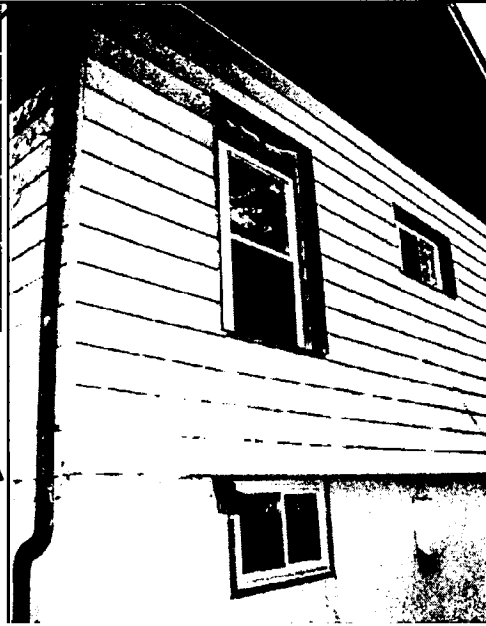
Basement Vinyl Replacement Windows Remain
