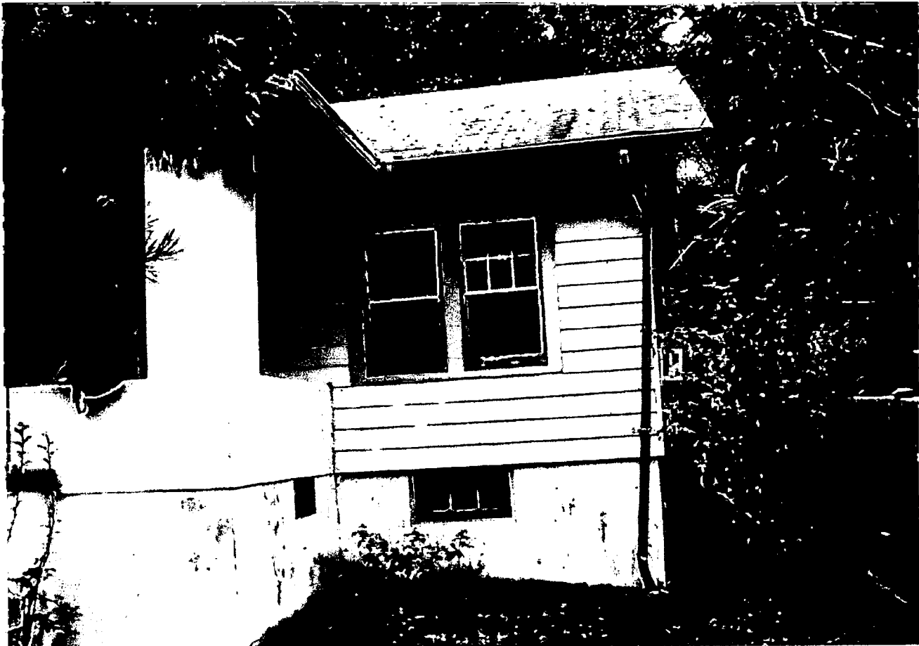
FRONT SIDE EXISTING VIEW
