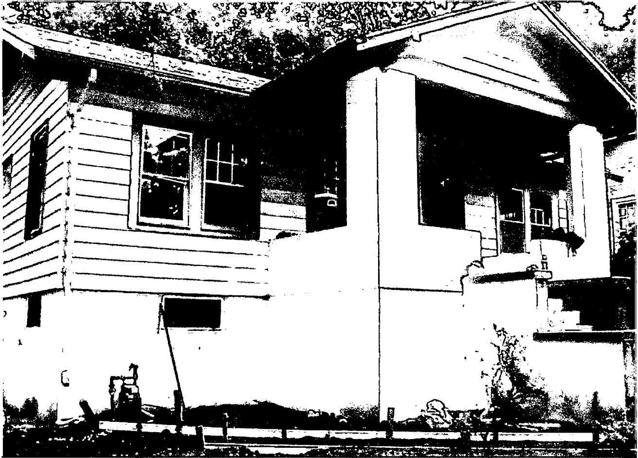
FRONT SIDE EXISTING VIEW
