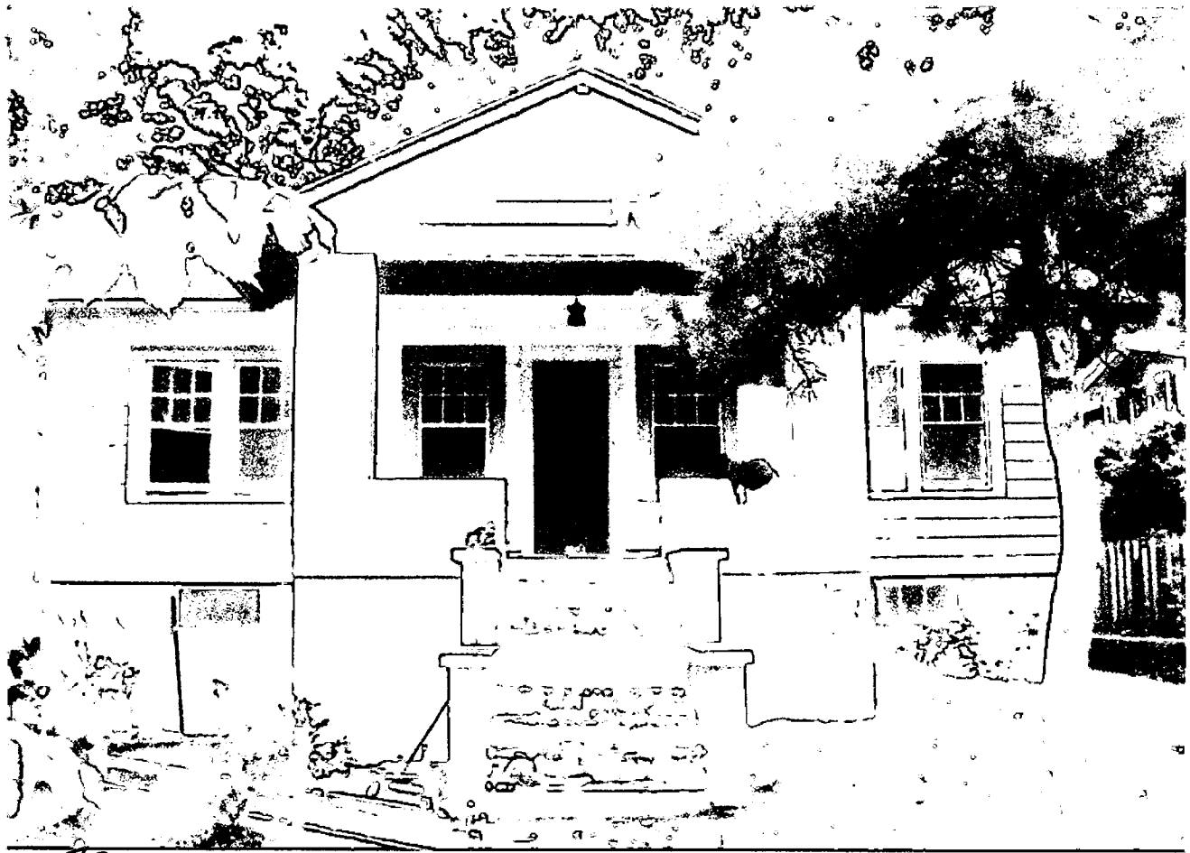
FRONT SIDE EXISTING VIEW
