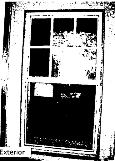
Remaining Wood Windows – Front Elevation
