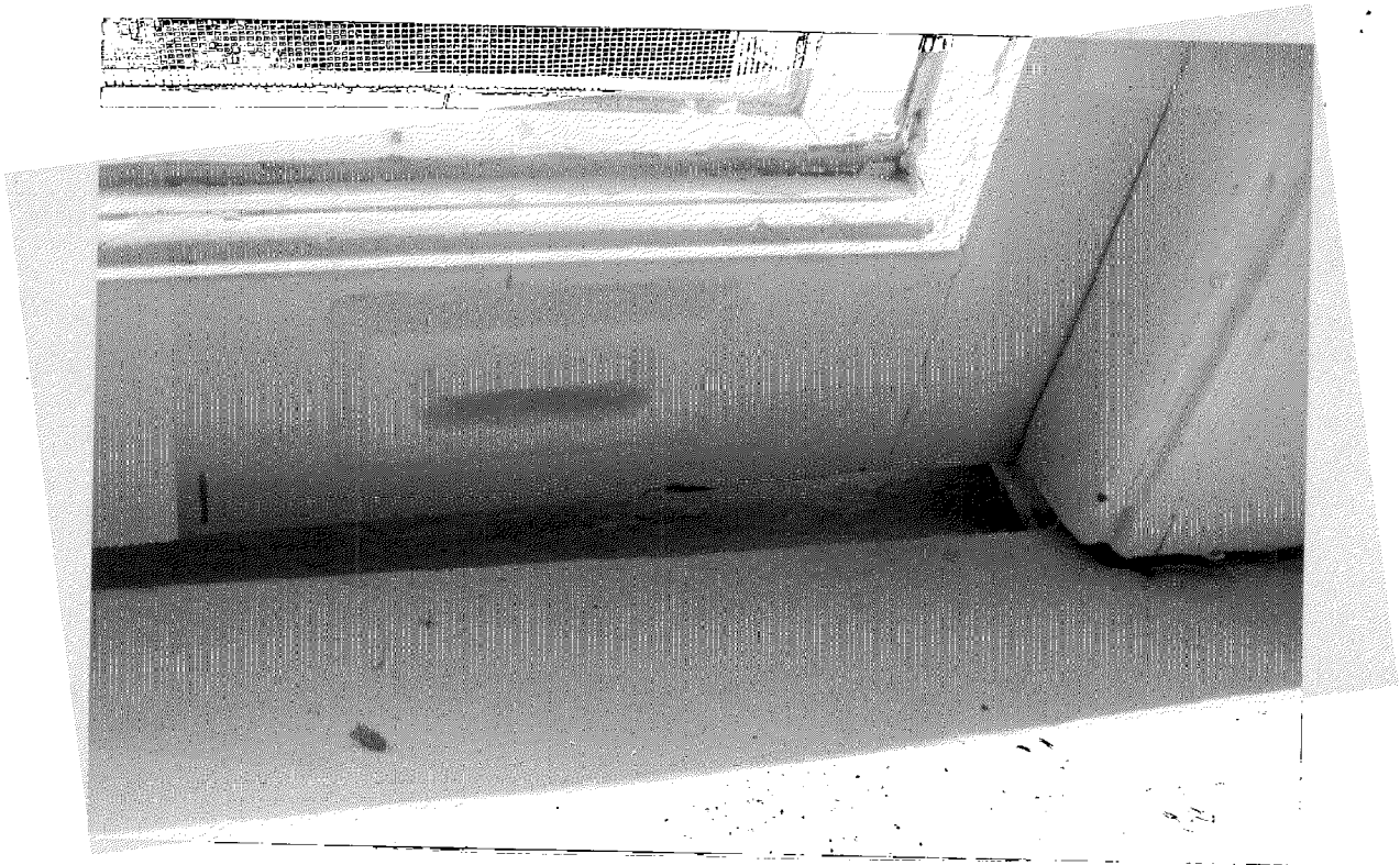
BOTTOM OF BOTTOM SASH IN CLOSED POSITION.
