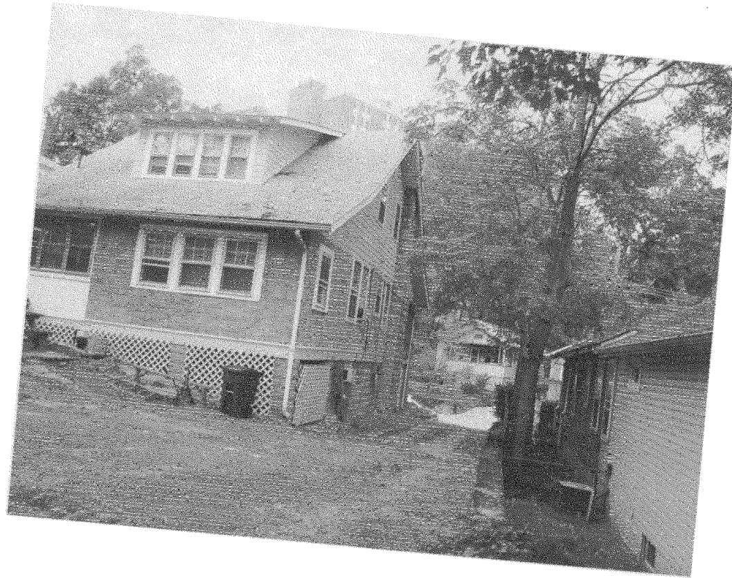
REAR OF 7004 Westmoreland Ave as shown from property edge of 7002.
