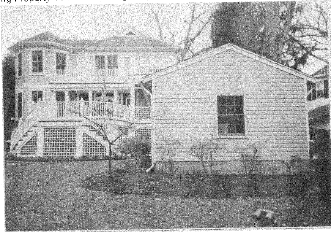
Detail: Back of garage; emergency generator will be placed behind garage
