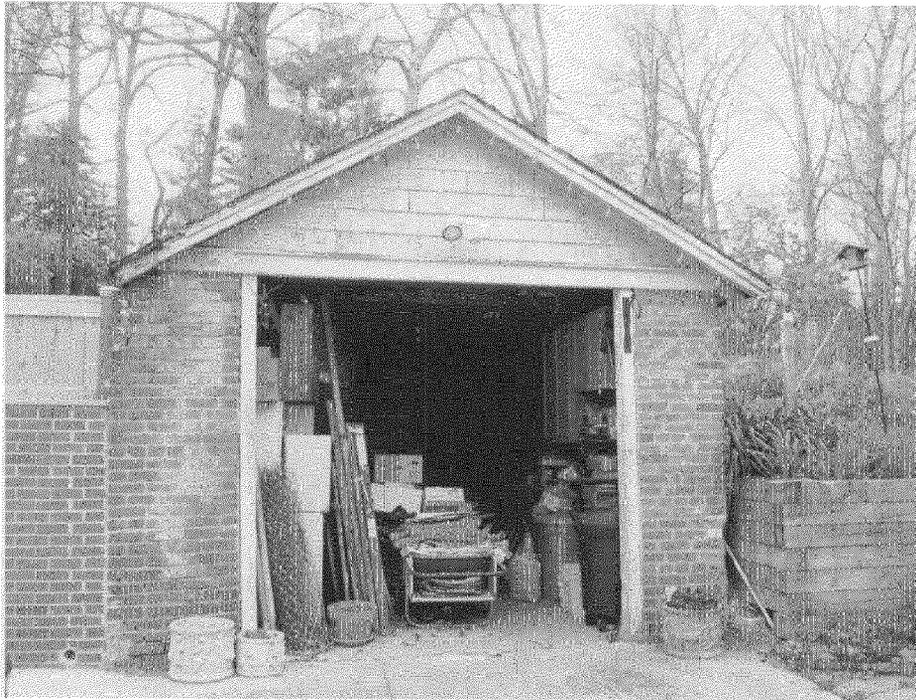
**Details: East façade of garage showing brick walls and shake shingle gable.**
