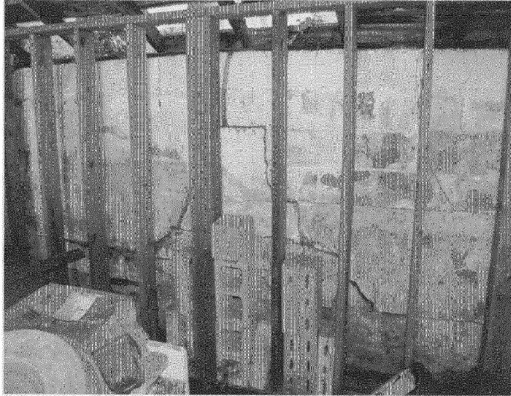
**Details: West wall interior detail showing replacement wall and cracks in cinder block wall. (View from B in Garage Photo Key)**
