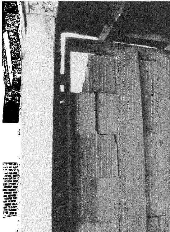
**Details: South wall interior detail showing replacement wall, crack in terracotta wall, and missing terracotta block. (View from A in Garage Photo Key)**
