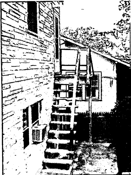
Detail: Side view, existing stairway. Instability and narrow platform and stair treads hinder usefulness and safety, also limit our ability to enjoy our outdoor space.
