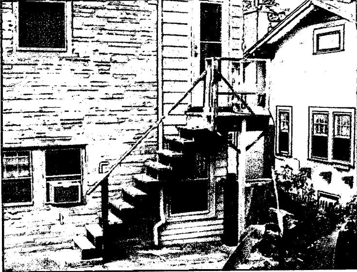
Detail: Existing platform and steps, leading from door off of our kitchen. Door is at the rear of the house. The door is on the main floor, basement floor is seen below.
