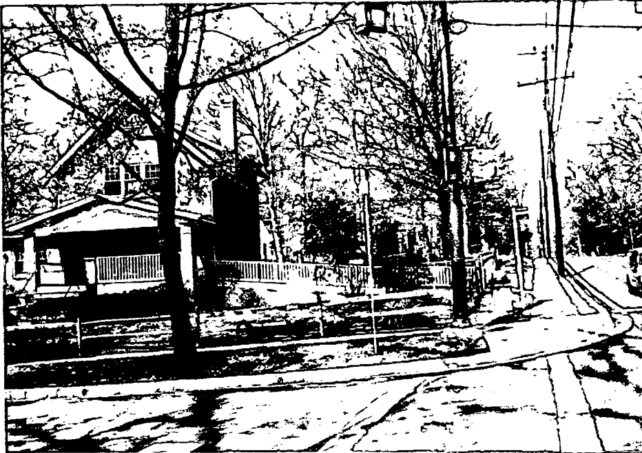
View from Takoma & Philadelphia Avenues
