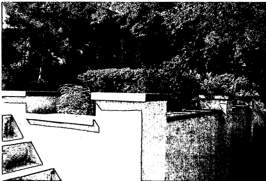
Detail: (7313 WILLOW) WALL STYLE WE WANT TO USE: DETAIL OF CONCRETE BODY W/ STONE TOPPERS
