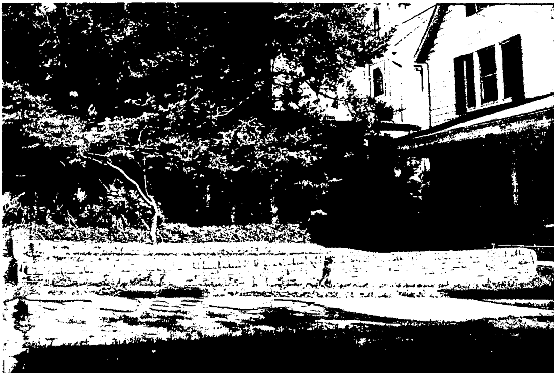
Detail: 402 Tulip Ave: BRICK WALL CONT' ALONG DRIVEWAY
