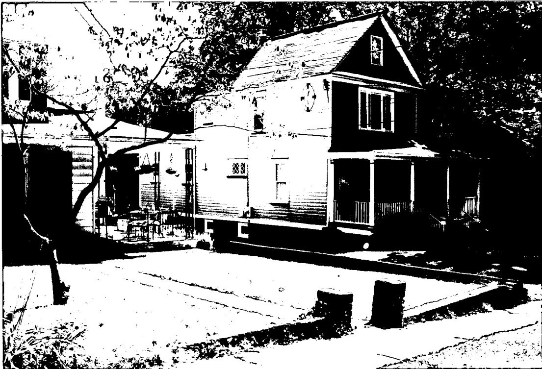
Detail: 402 Tulip Ave: BRICK WALL ON FRONT OF HOUSE
