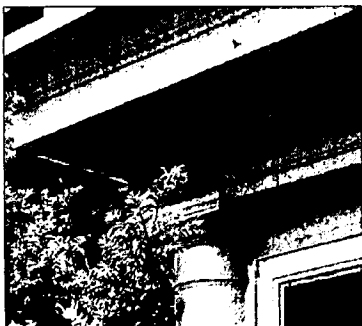
Porch enclosures that are attached to existing decorative porch elements such as this column can cause damage that is both difficult and costly to repair.
