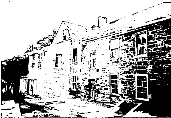
e.jpg South/West Elevation Section to be demolished has flat roof. Window will be saved.
