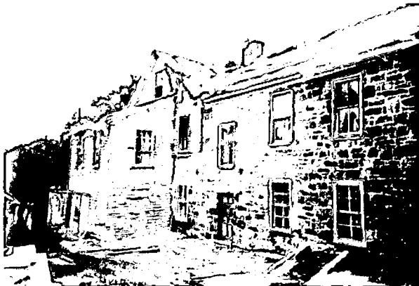
South/West Elevation Section to be demolished has flat roof. Window will be saved.
