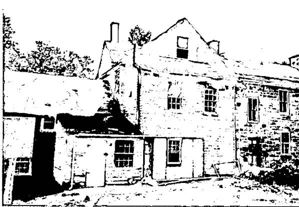
c.jpg Section of House to be Demolished Includes the one-story space and the two-story space immediately to its right. Both spaces have flat roofs that slope toward the photographer. Windows will be saved.
