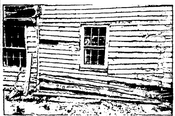
Detail of Structural Problems. Foundation is crumbling.
