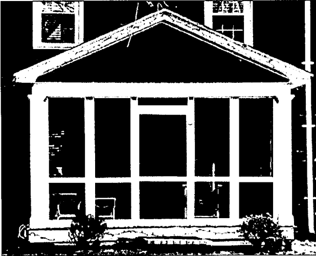
The large areas of screening on this porch make it appear more like a porch than an enclosed room. It is recommended that the white screen enclosure framing be painted a darker color, similar to the screen color, to minimize its visibility.
