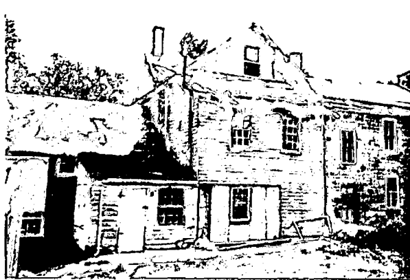
Section of House to be Demolished Includes the one-story space and the two-story space immediately to its right. Both spaces have flat roofs that slope toward the photographer. Windows will be saved.
