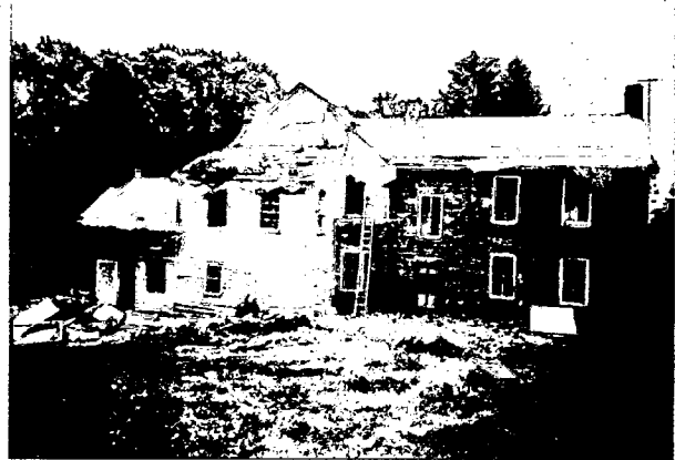
b.jpg West Elevation of Farmhouse
