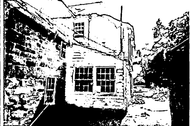
North Elevation of Section to be Demolished Windows will be saved.
