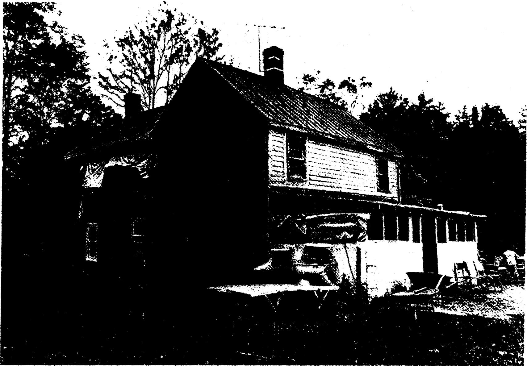
Figure 17. Jones-Hall-Sims log house, Jonesville. Probably built in 1874, this was the home of Richard Jones, who helped found the Jonesville community. Changes include the addition of a two story frame block to the back length, weatherboards over the logs, and a shed porch to the front. In 1896, Levin Hall purchased the house, and four generations of his descendants live there today.
