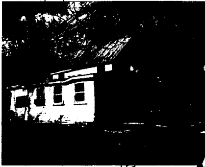
Jones-Hall Hse (c1874) 18425 Jonesville Ter Condemned
