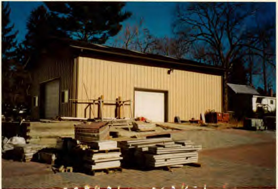
Butler Building Install Horizontal Siding French Doors on Front
