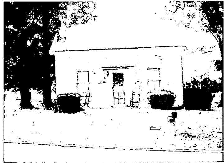
Picture 16: Picture of house (commercial zoning) at 15120 Barnesville Road
