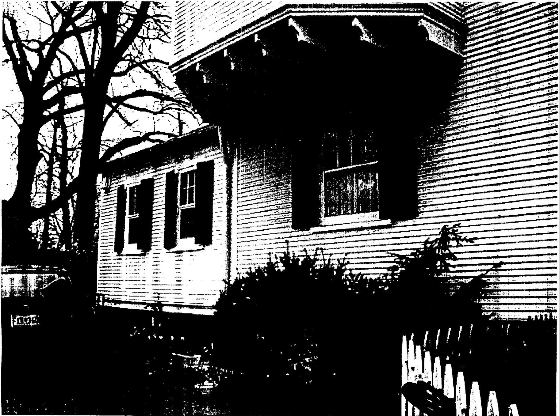
PORTION OF EAST ELEVATION SHOWING 2ND FL. CANTILEVERED BAY AND 1915 ADDITION
