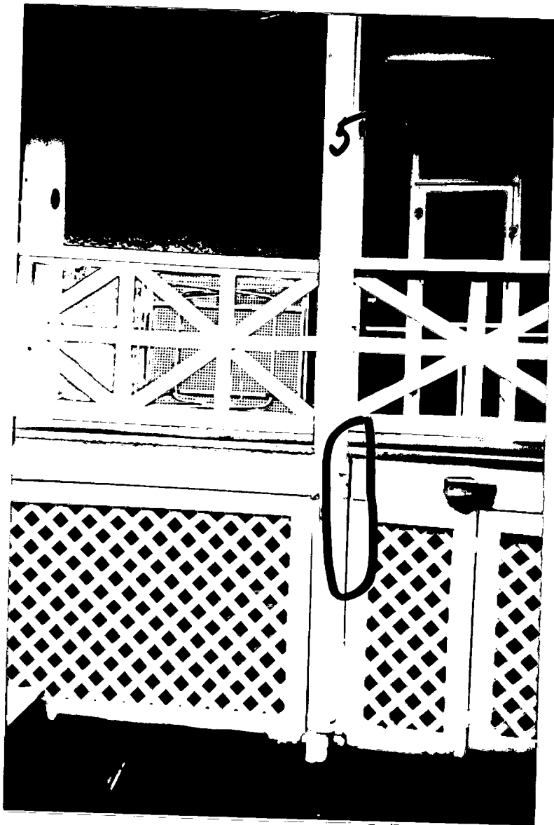
CRACKS IN PORCH
