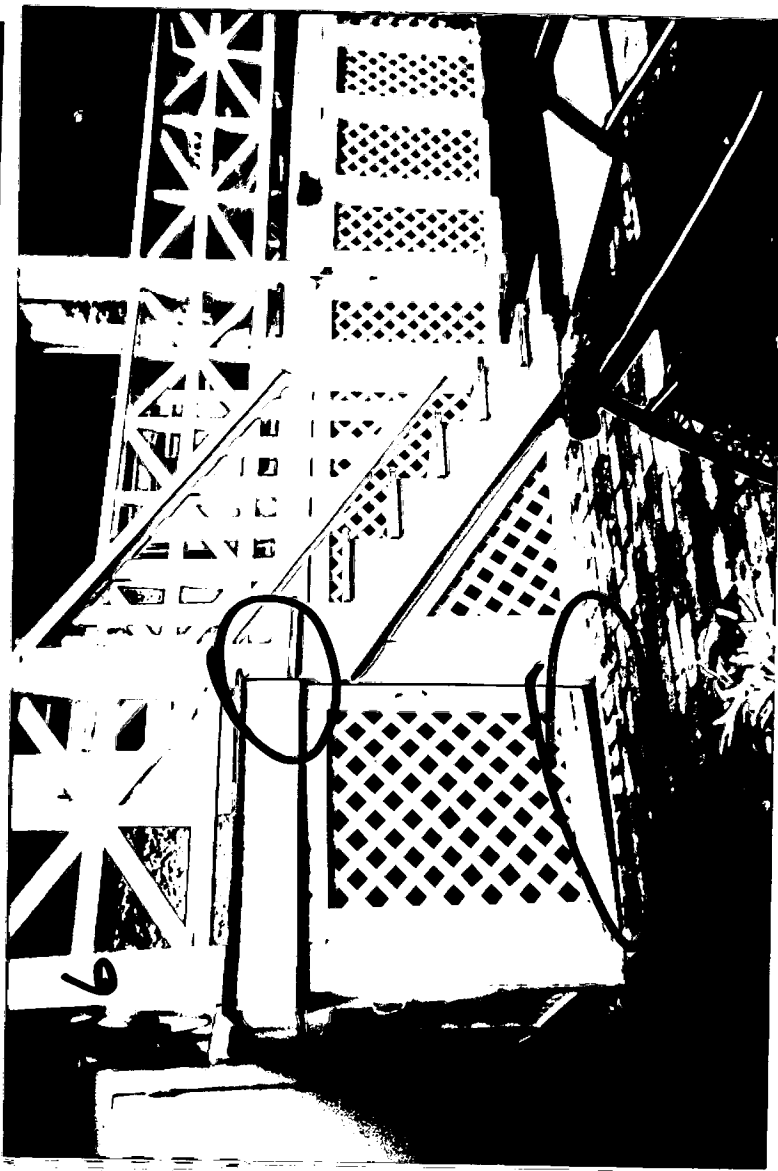
CRACKS IN PORCH
