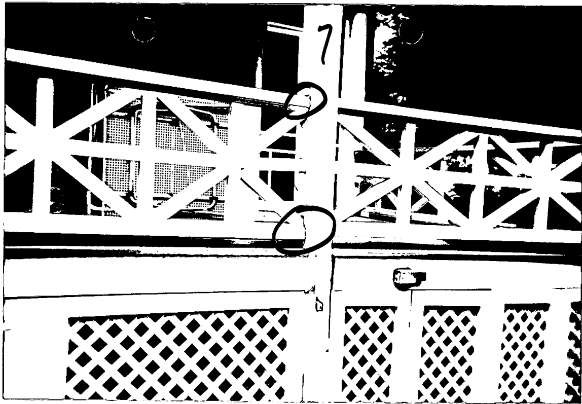
CRACKS IN PORCH
