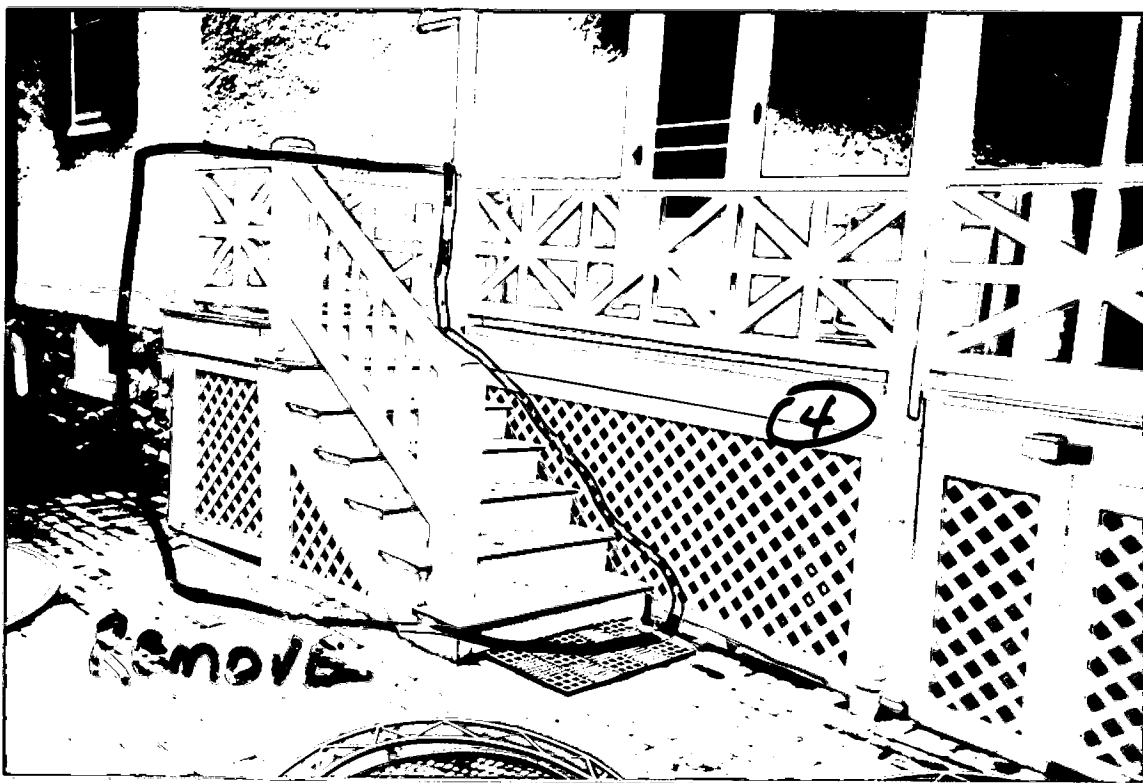
EXISTING PORCH + STEPS
