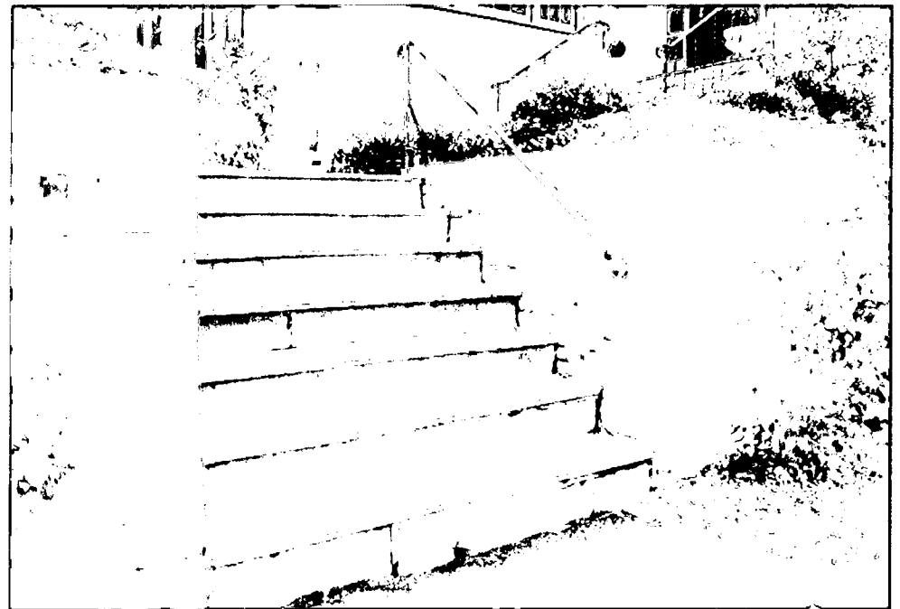
existing steps to be removed & replaced.
