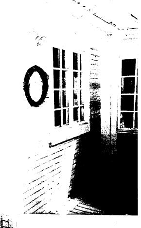
Window on west side will be swapped with door on north side. A new 5-0x6-8 double door will be installed on west side.
