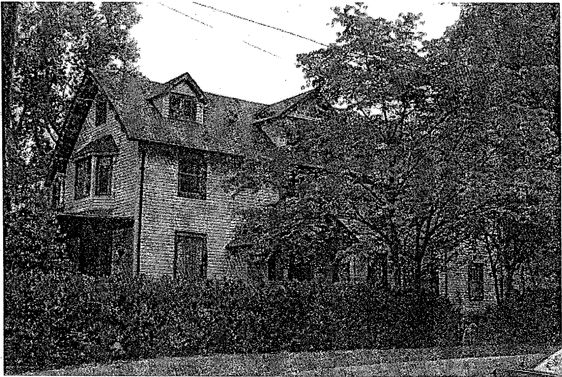
Front elevation (southwest) from public right-of-way
