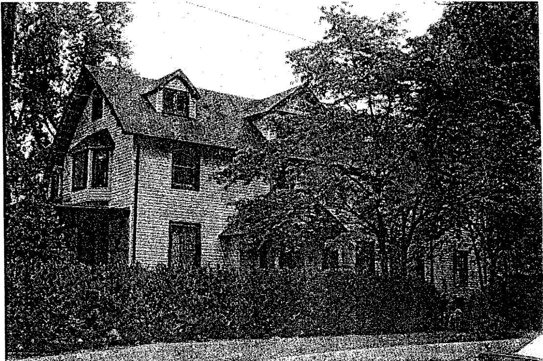
Front elevation (southwest) from public right-of-way
