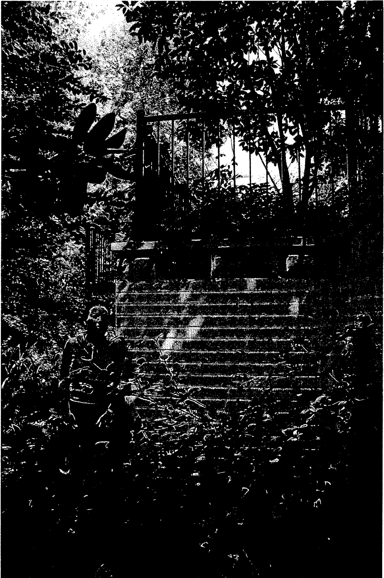
Our view of the Holverson/Smith retaining wall.
