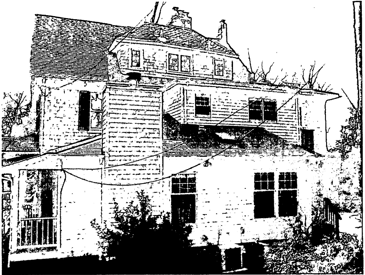
Elevation east side (toward 3 West Lenox) 5 W. Lenox St.
