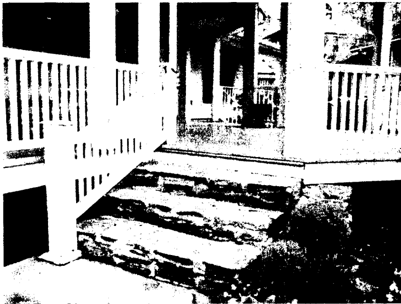
Front steps to porch. Wood handrail (to the left) will be removed and an iron rail Will be installed to the right. (above)
