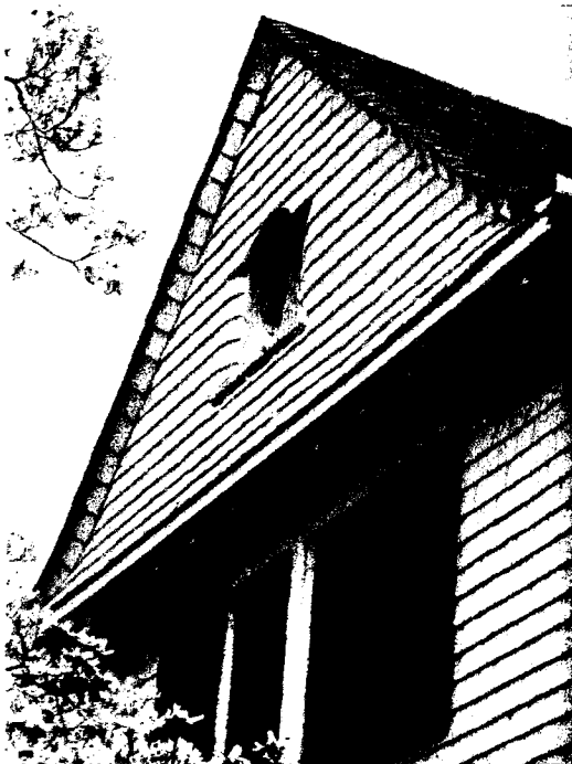
Close-up of fan in gable; shakes at top of the opening will be restored to square, and the curved sides and sill will be retained as is.
