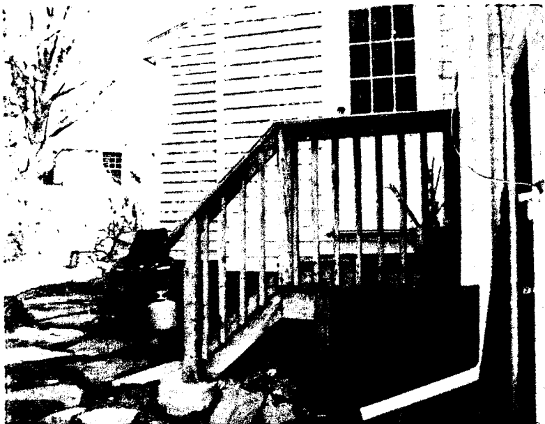
Slope at bottom of back stairs where stone steps would be added for safety and to accommodate grade change to back walkway
