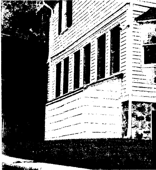
View of lean-to shed from street
