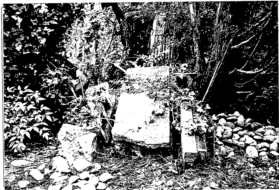
Detail: East side wall that fell
