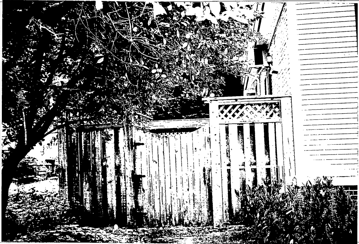
Detail: East side yard as seen from front of property
