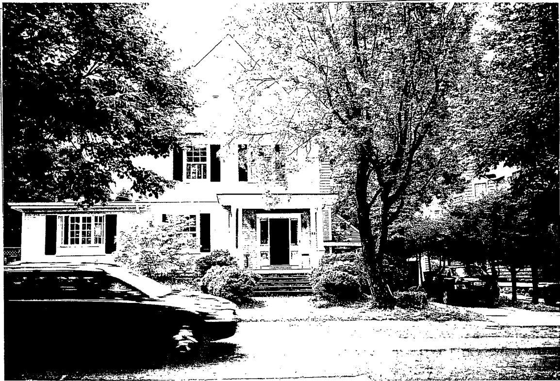
Detail: Front & E. Lenox with attention to west side
