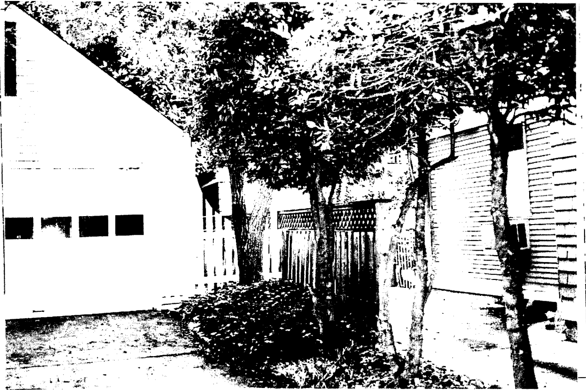
Detail: Unpainted fence to be removed. New fence to commence at white picket fence with lattice. New wire to harmonize with existing picket fence.
