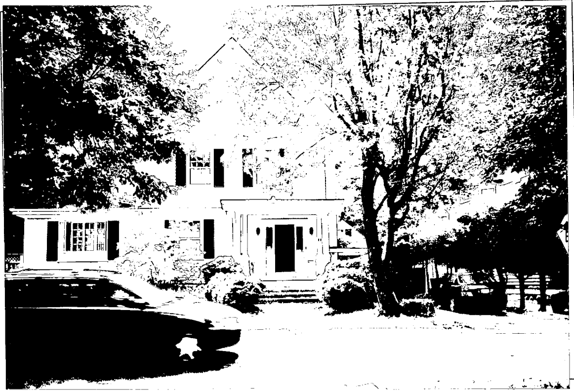
Detail: Front, 8 E. Lenox with attention to west side
