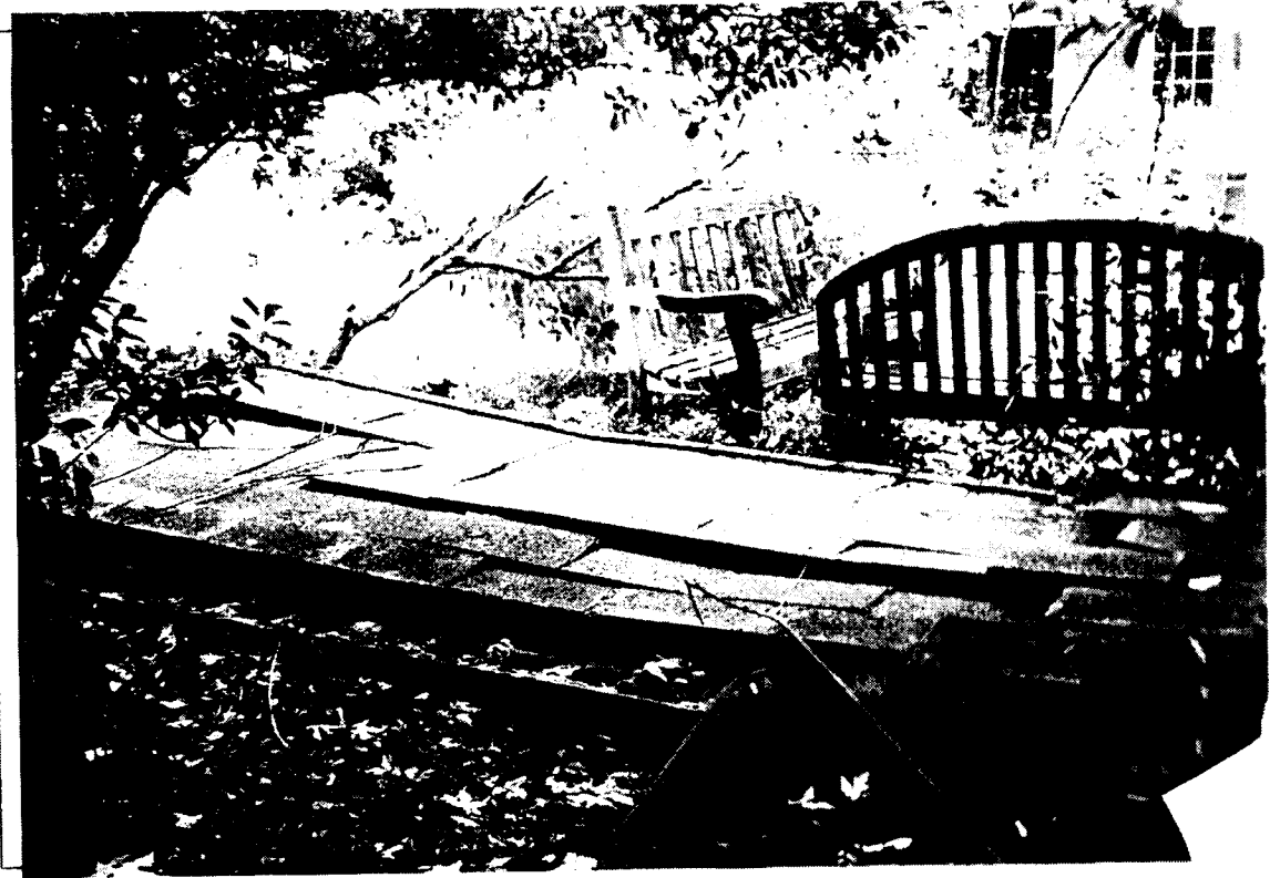
Detail: East side wall that fell seen from lot corner
