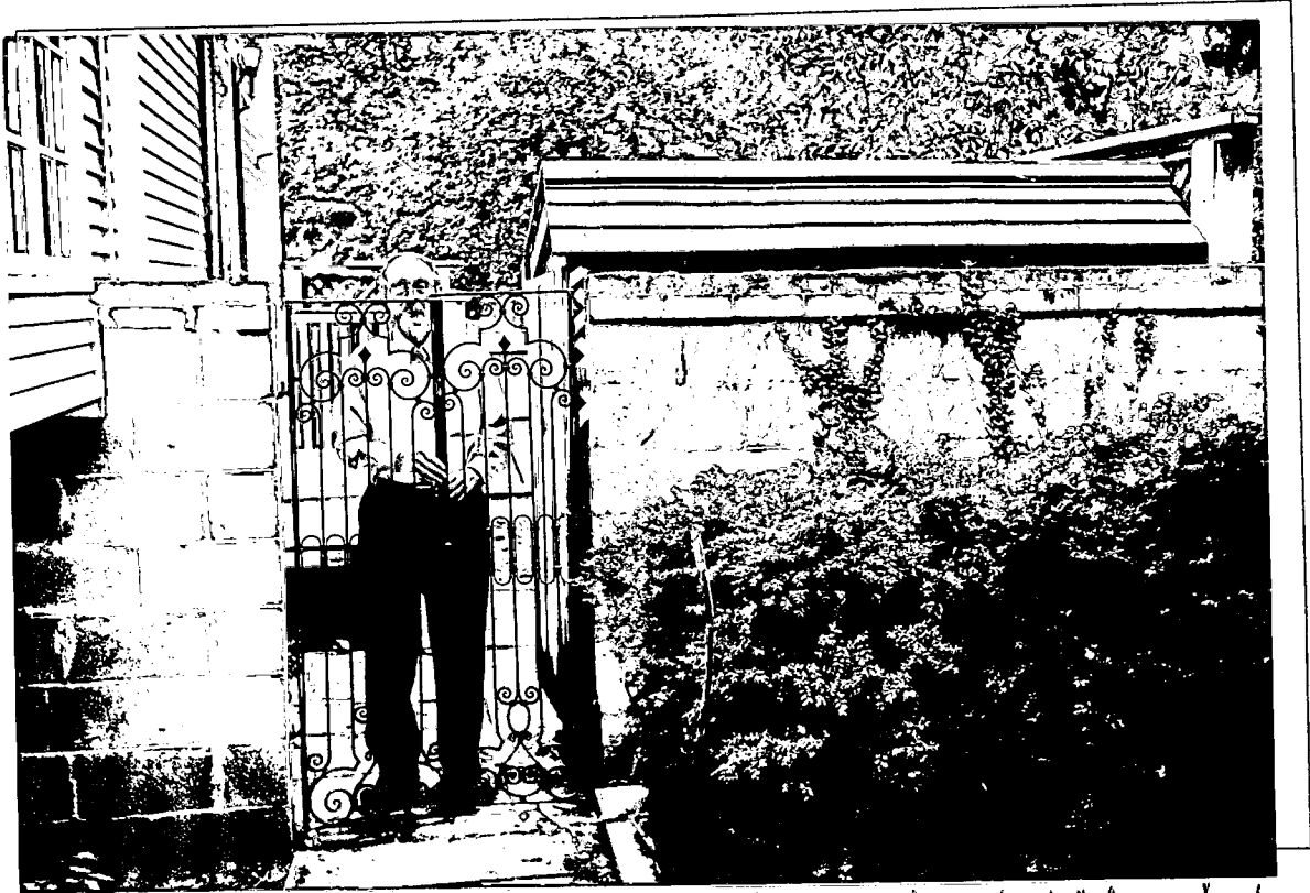
Detail: East side wall with ornamental iron gate at right angle to proposed ornamental aluminum fence
