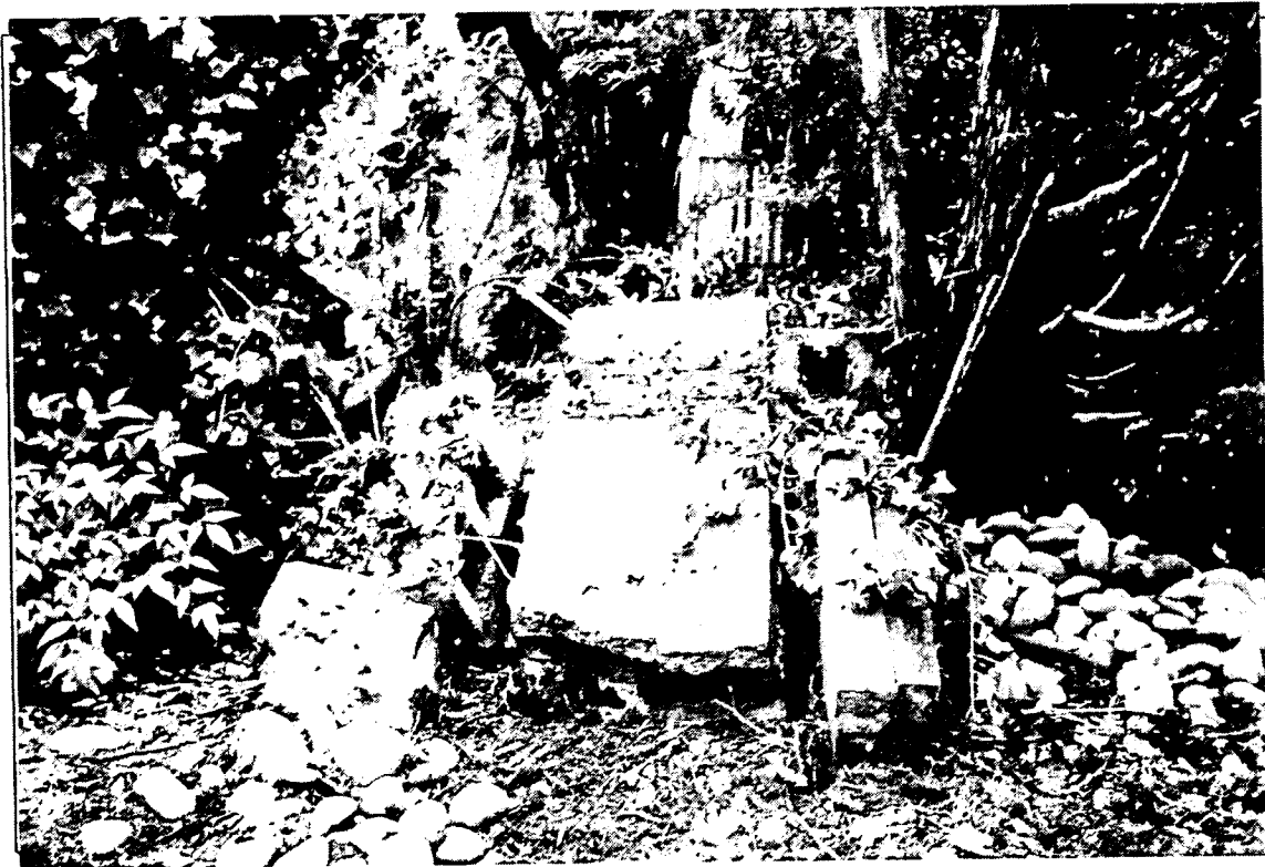
Detail: East side wall that fell
