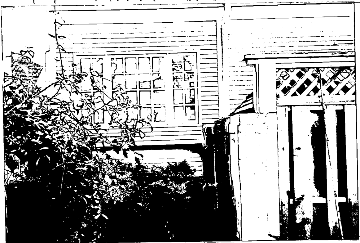
Detail: East side where fence will abut wall as seen from east neighbor (6 E Lenox)
