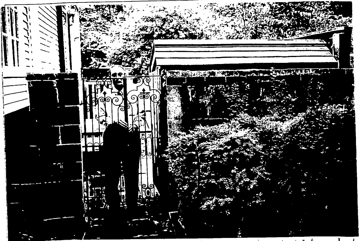
Detail: East side wall with ornamental iron gate at right angle to proposed ornamental aluminum fence
