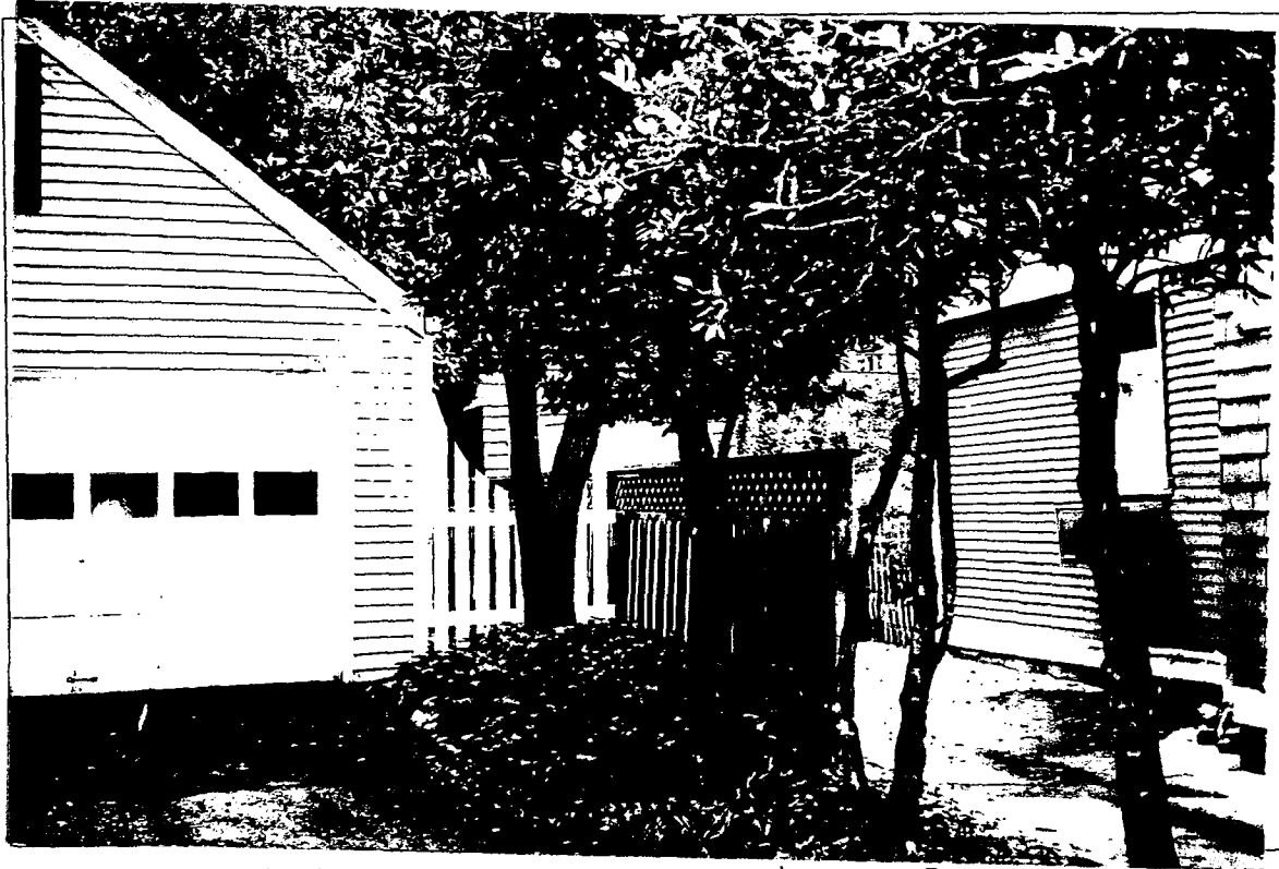
Detail: Unpainted fence to be removed. New fence to commence at white picket fence + run south. New fence to harmonize with existing picket fence.
