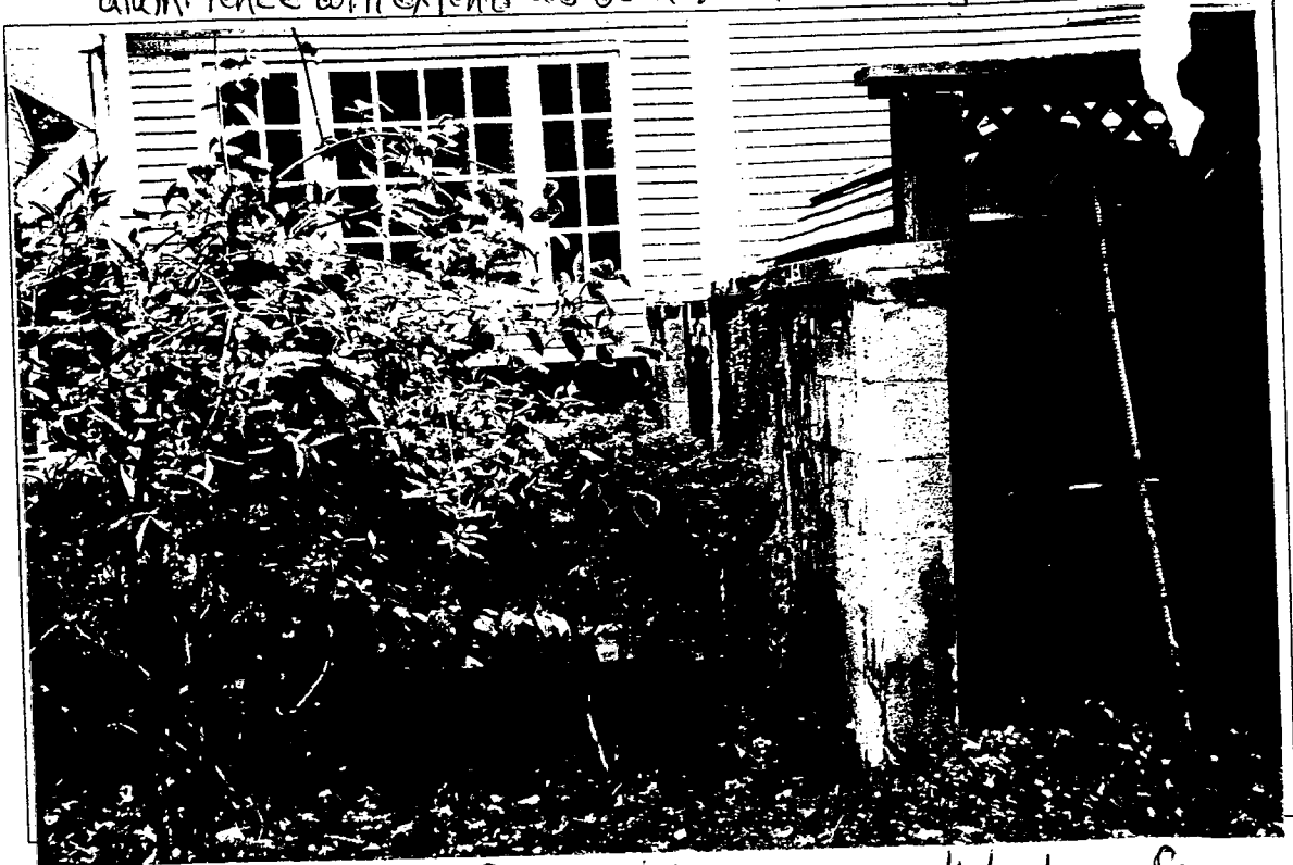
Detail: Again, point from which ornamental alum. fence will start - toward north of property - as seen from 6E Lenox
