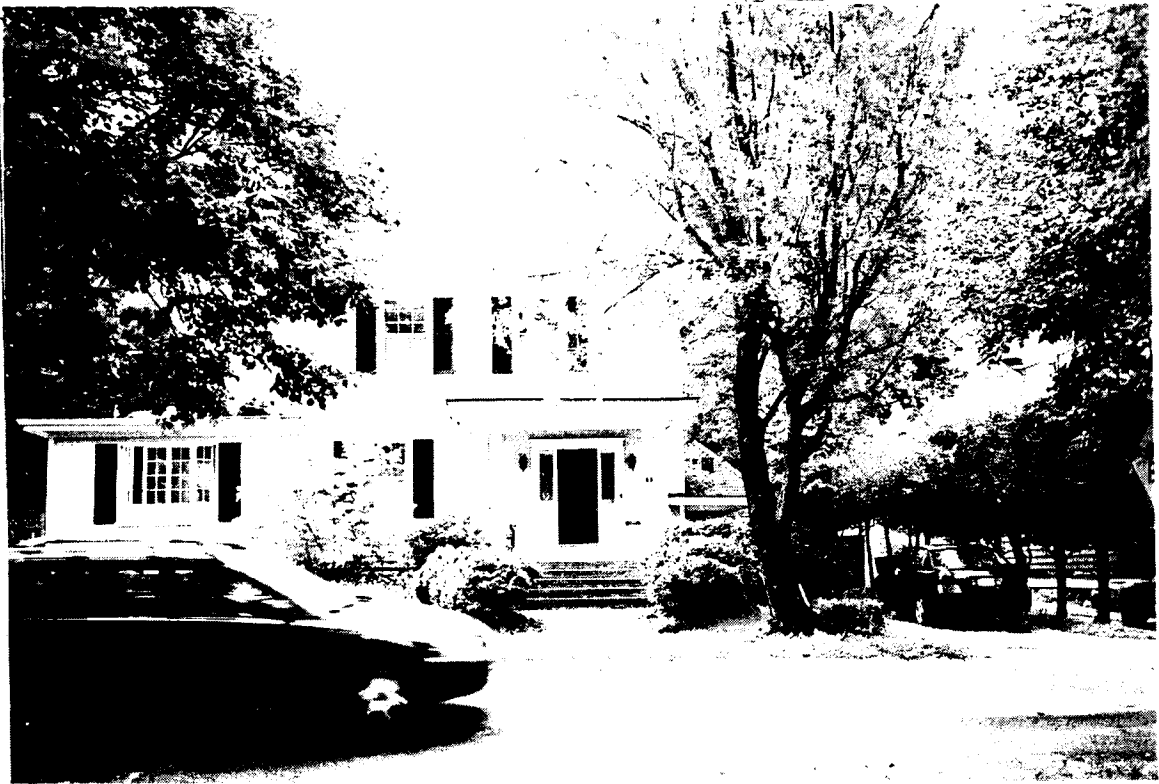
Detail: Front, S.E. corner with attention to west side
