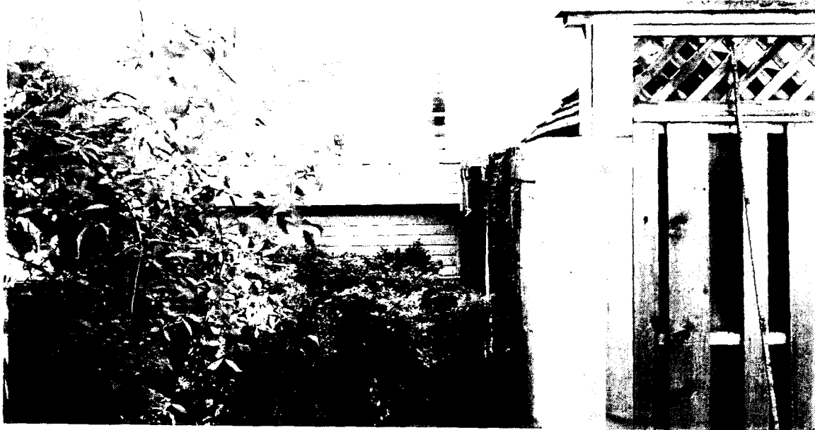
Detail: East side where fence will abut wall as seen from east neighbor (G.F. Linnex)
