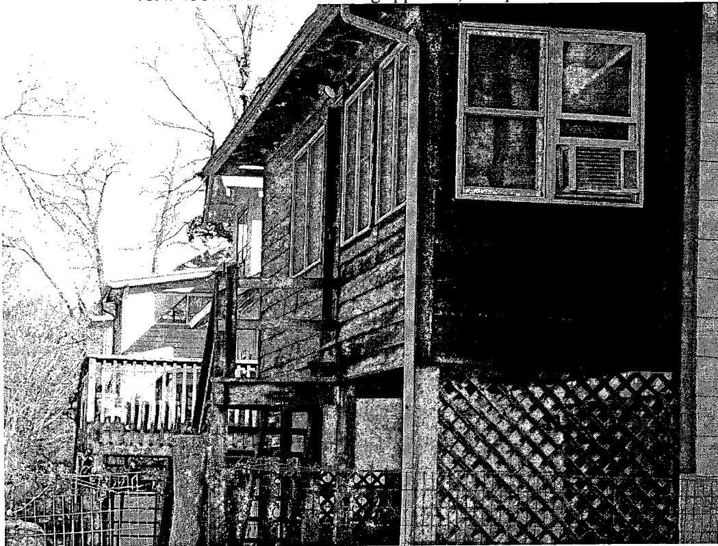
View of adjacent decks and steps at rear of houses to the immediate east
