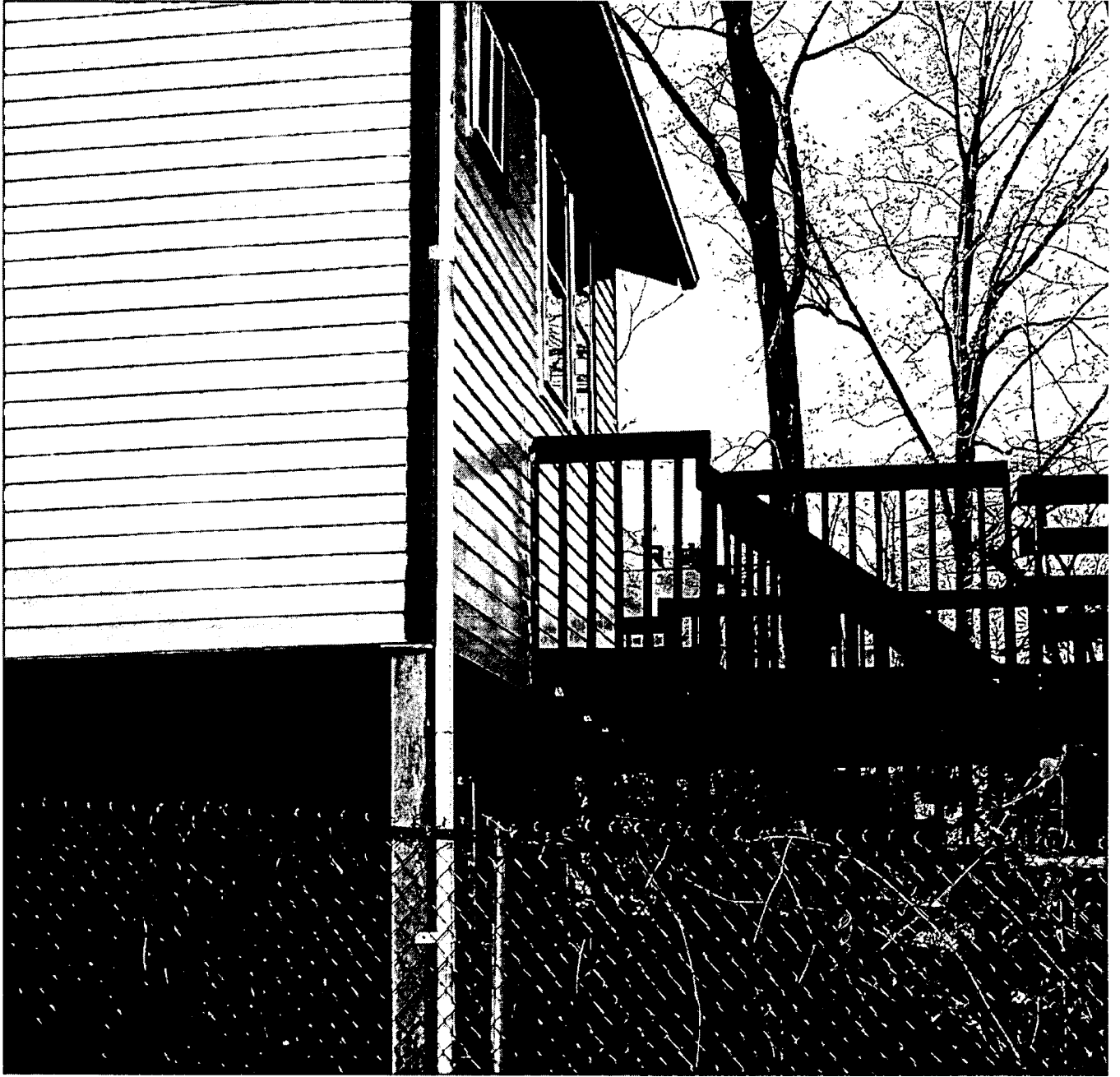
View of deck to the immediate west
