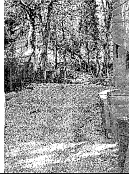
Current gravel extension beyond 30' asphalt paving
