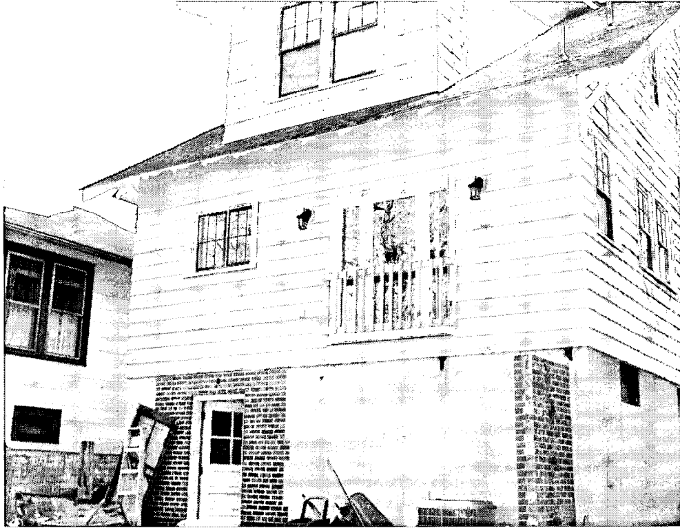
View of rear elevation showing approved, new patio door
