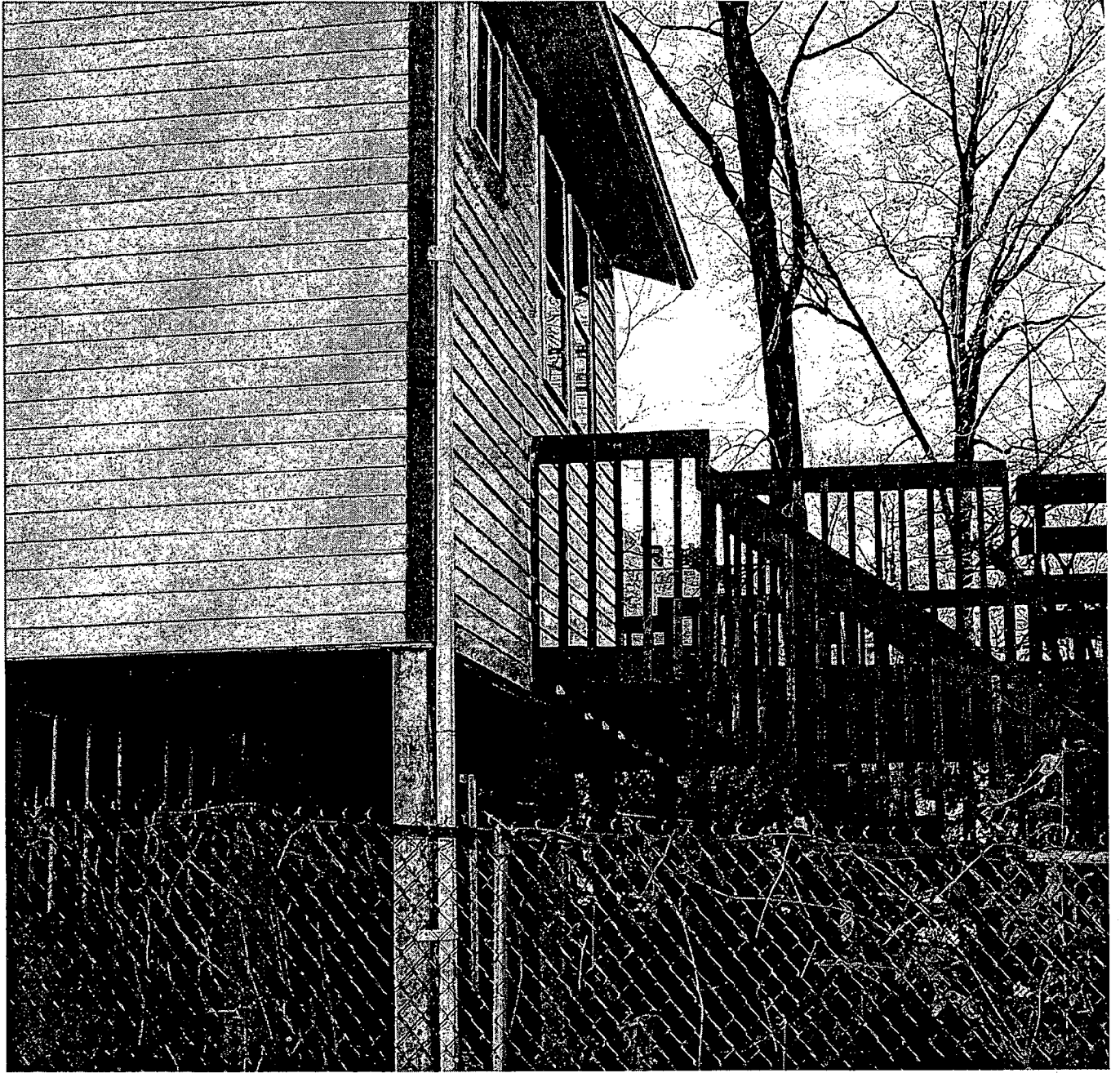
View of deck to the immediate west
