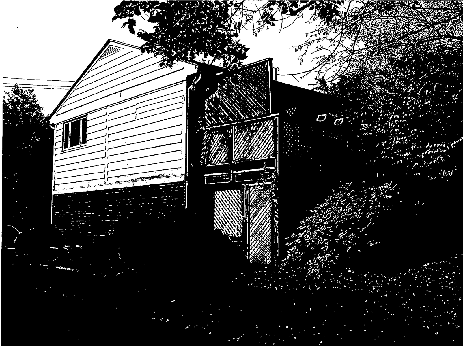
Sen Residence 7512 Carroll Avenue Side/Deck View from northwest
