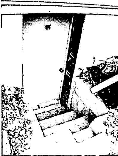
Replacement door and areaway stairs
