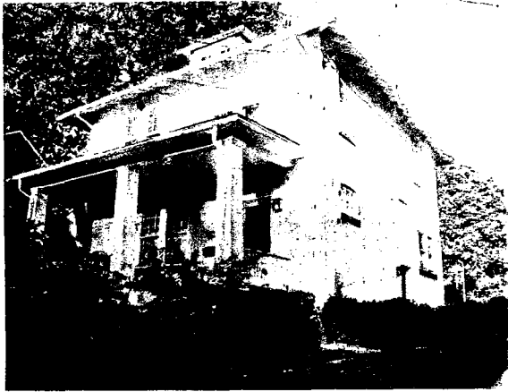
View of 7136 Carroll Ave. from the front sidewalk
