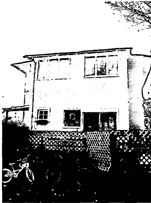
Views of rear addition showing existing aluminum sliding door and aluminum casement windows above
