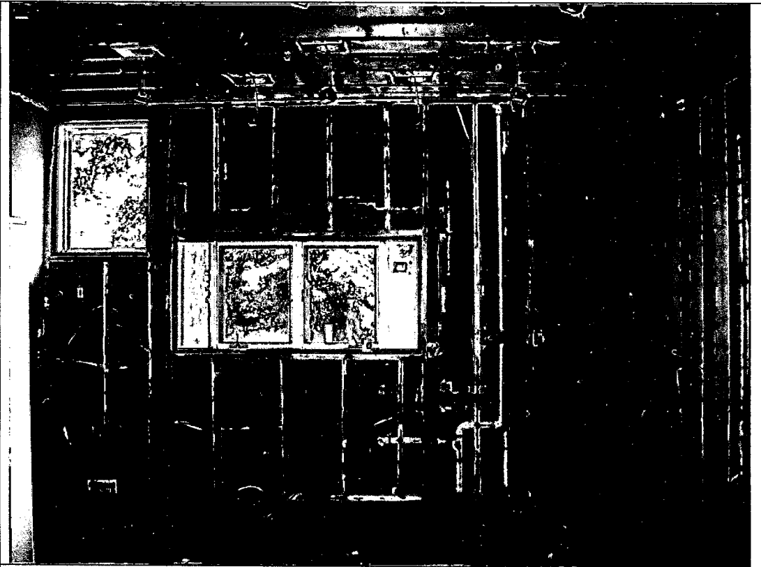
Back wall – Inside view
