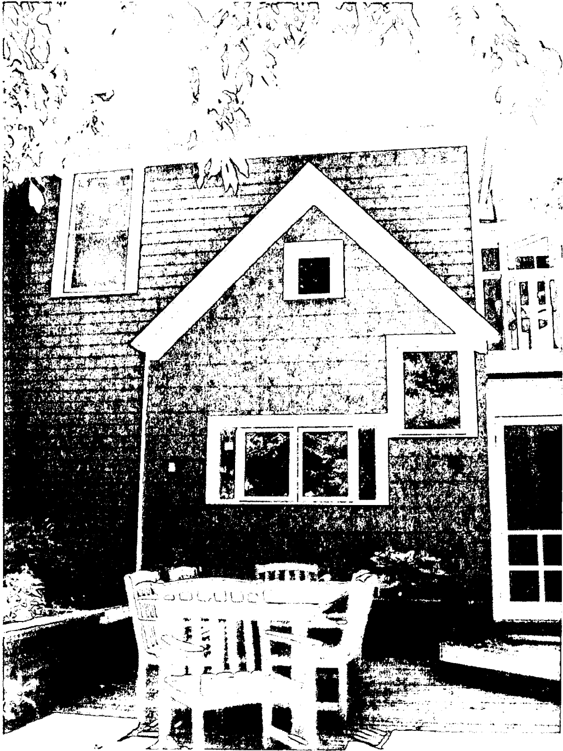
Back wall – Out side view
