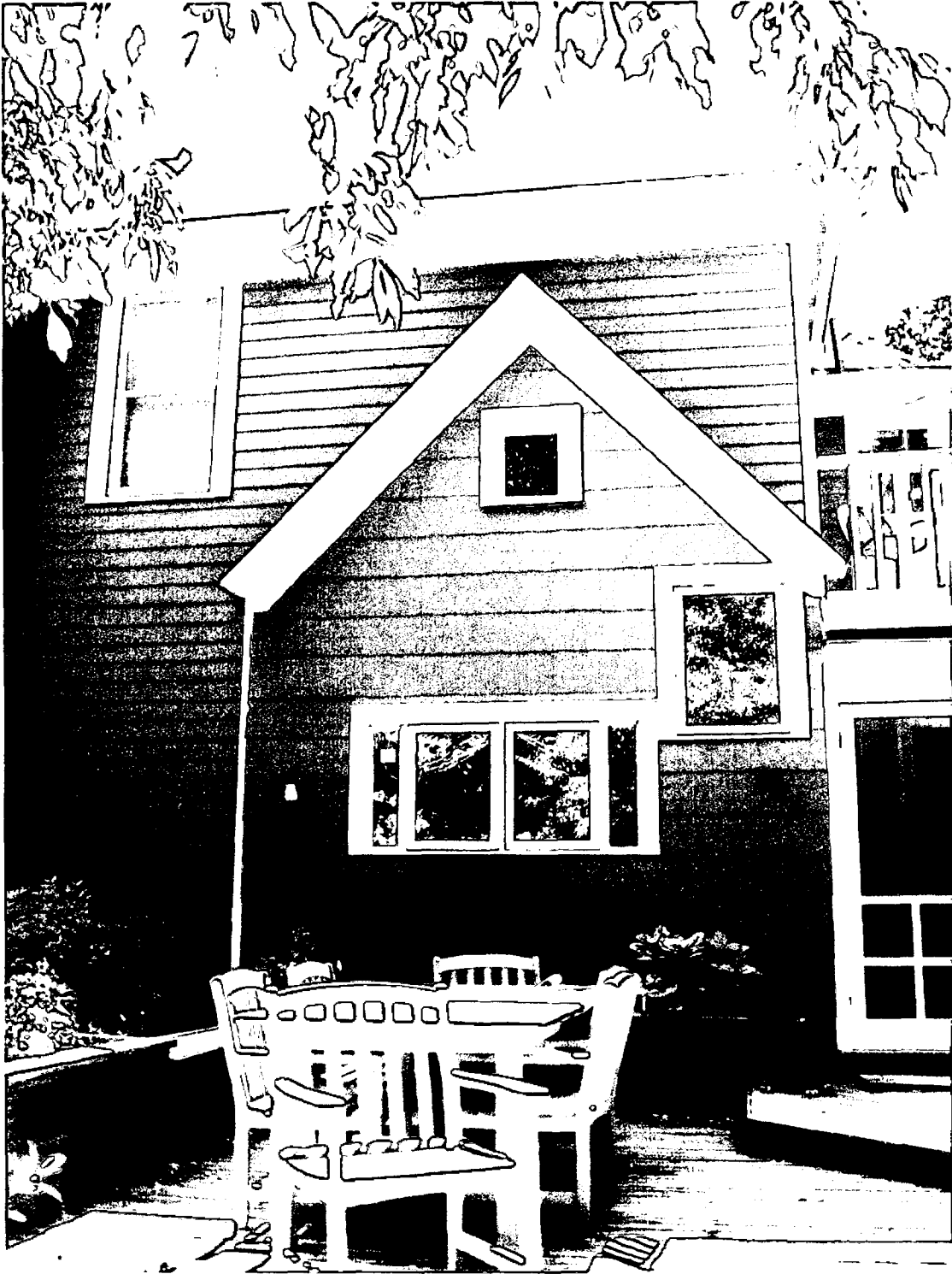
Back wall – Out side view
