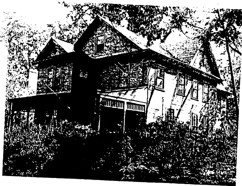
WEST (FRONT) ELEV - EXISTING VIEW FROM CEDAR STREET
