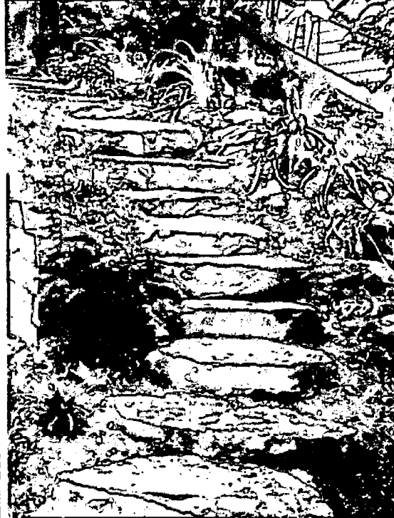
Boulder Steps Set in Ground
