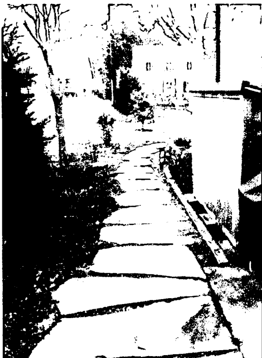
Irregular Pennsylvania Flagstone Set in Masonary Sand
