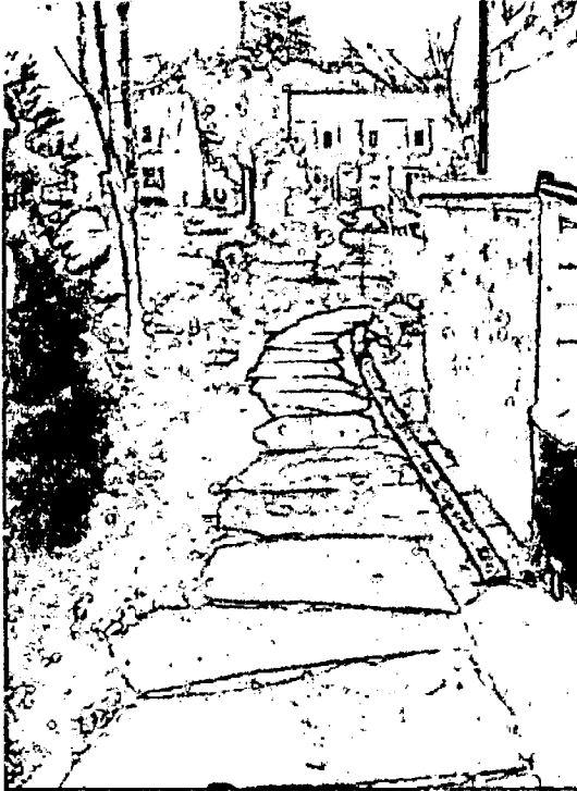
Irregular Pennsylvania Flagstone Set in Masonry Sand
