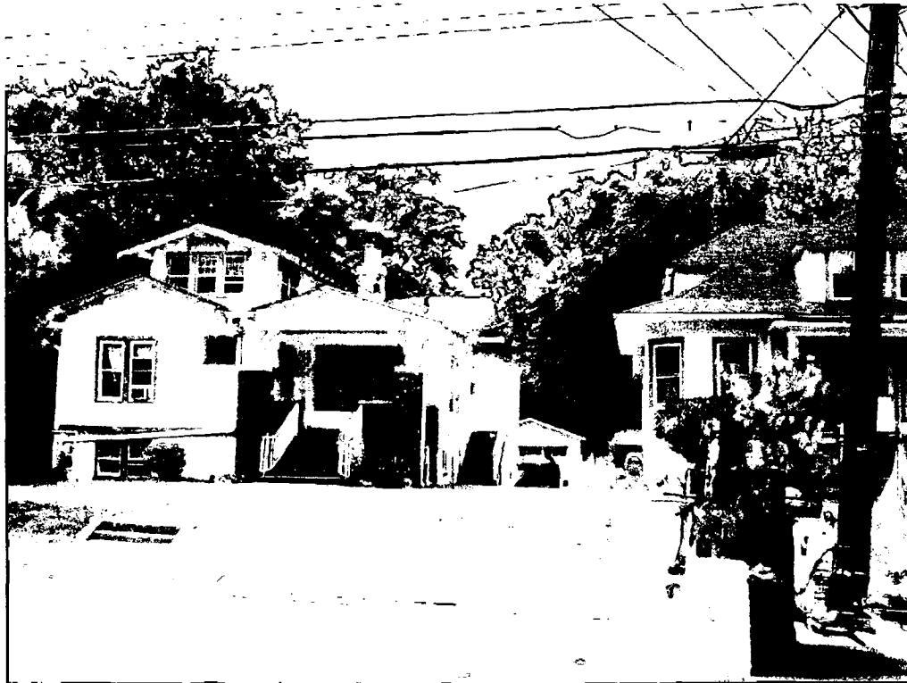
NEIGHBORHOOD PRECEDENT- View from Street of garage in rear yard of 7126 Carroll Ave.
