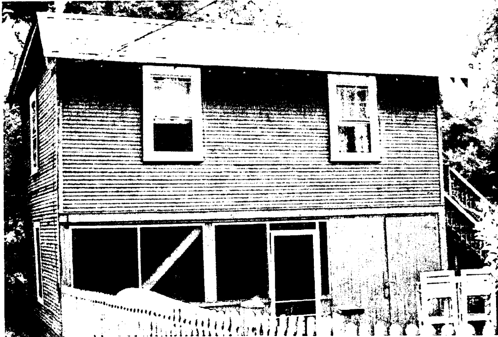
7123 CARROLL AVE. 2-STORY NON-HISTORIC STRUCTURE DEMOLISHED Request for retroactive approval to remove 2 story non-historic frame structure located in rear yard behind existing residence. Notice how left wall is canted.
