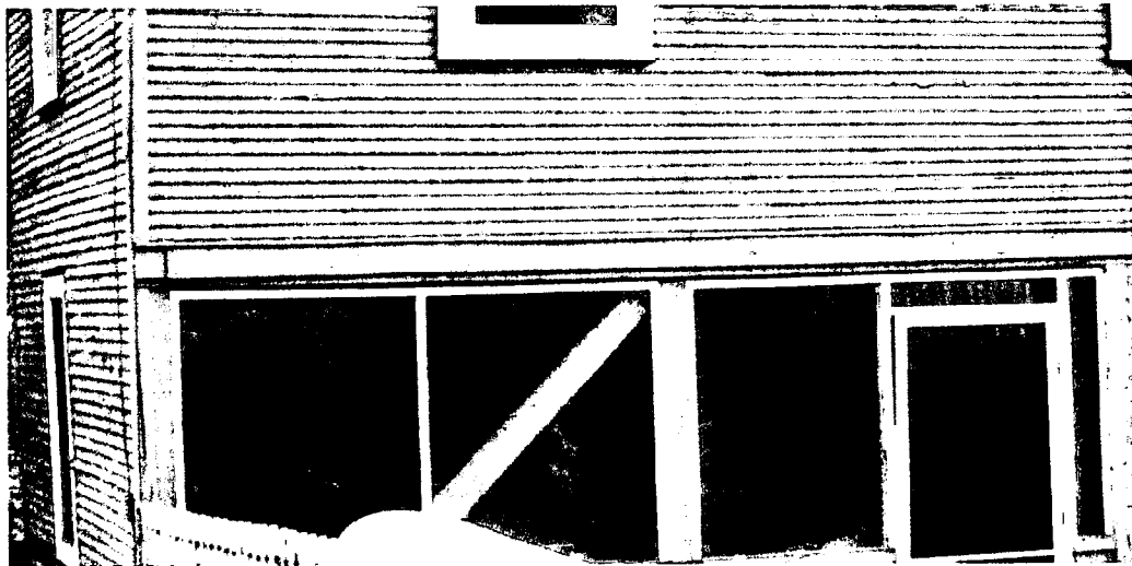
7123 CARROLL AVE. 2-STORY NON-HISTORIC STRUCTURE DEMOLISHED Request for retroactive approval to remove 2 story non-historic frame structure located in rear yard behind existing residence – Detail of bracing used to minimize building movement in wind.
