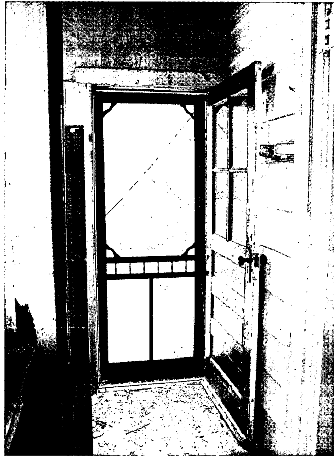
Interior view of door with historic screen (being replaced)
