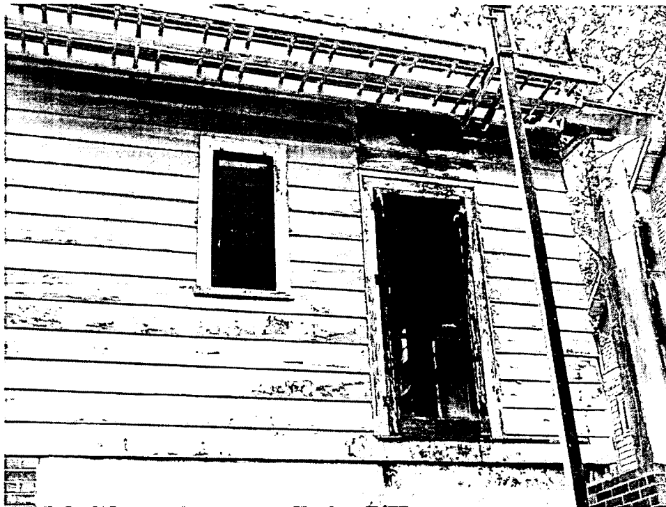
Door and 1/1 double hung window on the rear
