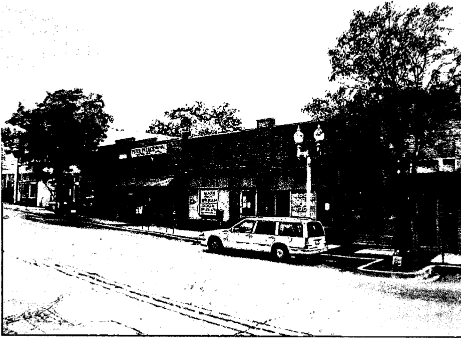
View of adjoining properties from across Carroll Avenue
