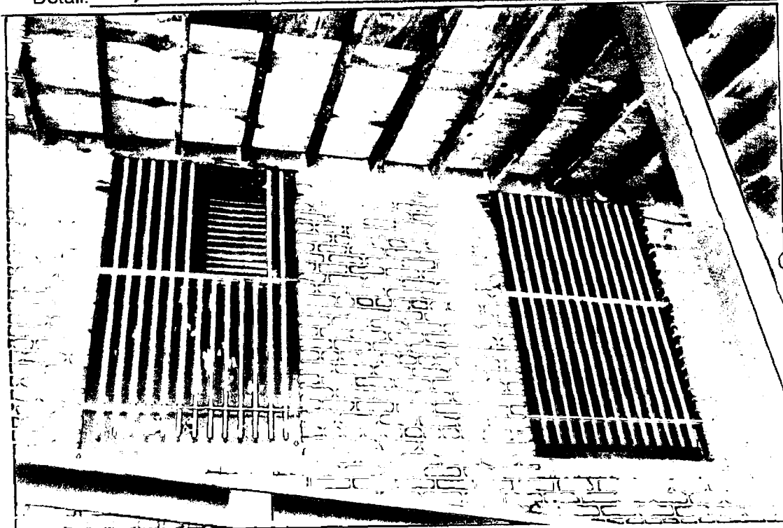
Detail: 2 WINDOWS TO BE REPAIRED
