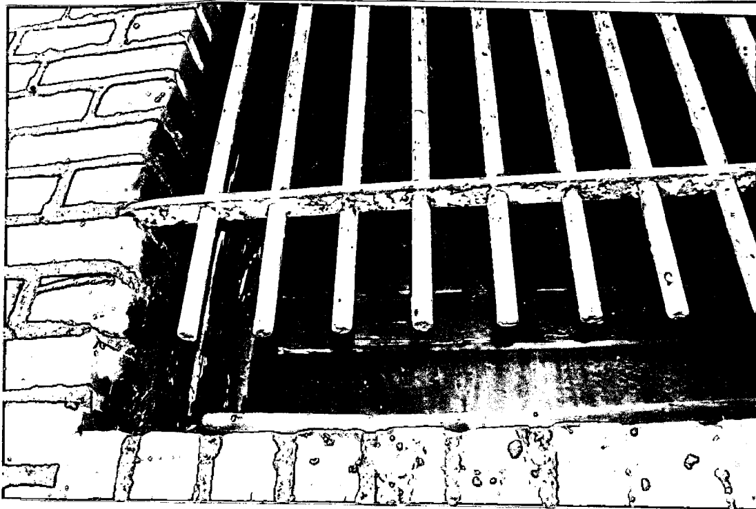
Detail: RIGHT WINDOW (FROM REAR) NOTE NOTED JAMB
