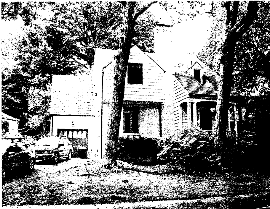
Front (east) side of house. 4 windows to be replaced - one downstairs and two upstairs, + one basement This side faces the street.
