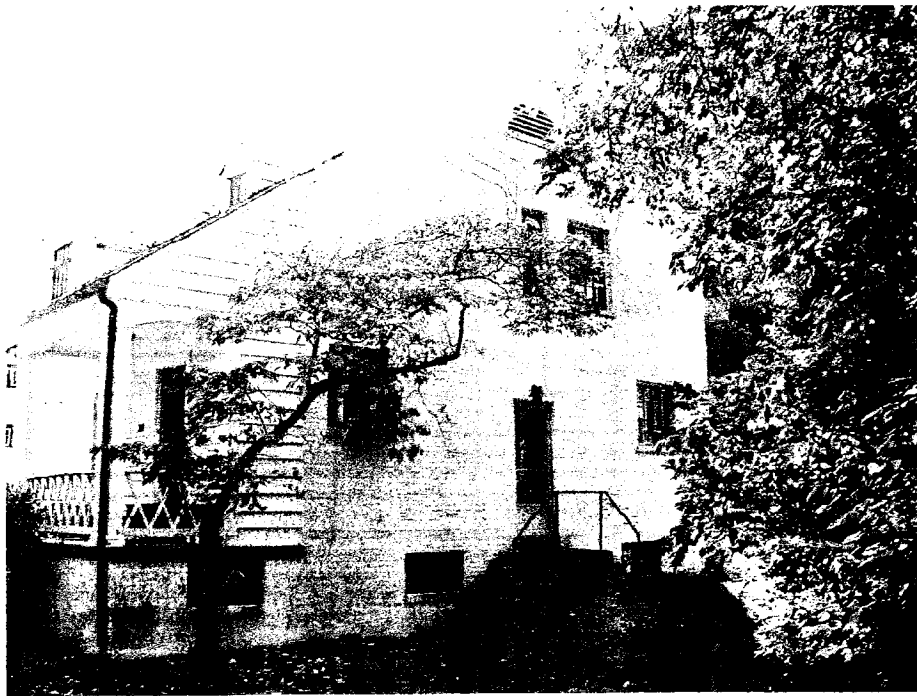
North side of house, visible from street. 7 windows to be replaced - 2 upstairs, 2 downstairs (including one w/window A/C unit) and 3 basement. Visible from neighbor's house.
