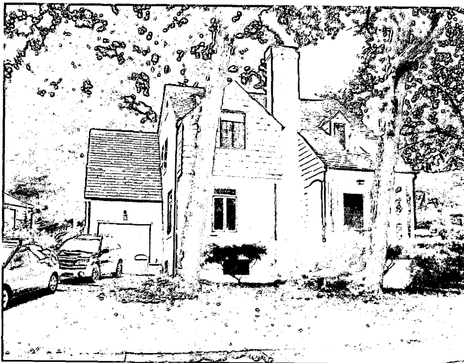
Front (east) side of house. 4 windows to be replaced - one downstairs and two upstairs, + one basement This side faces the street.
