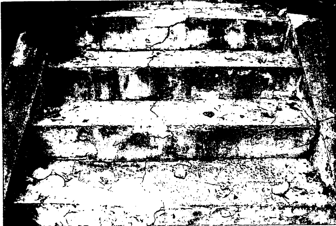
Detail: Front staircase, close-up (bottom stairs)
