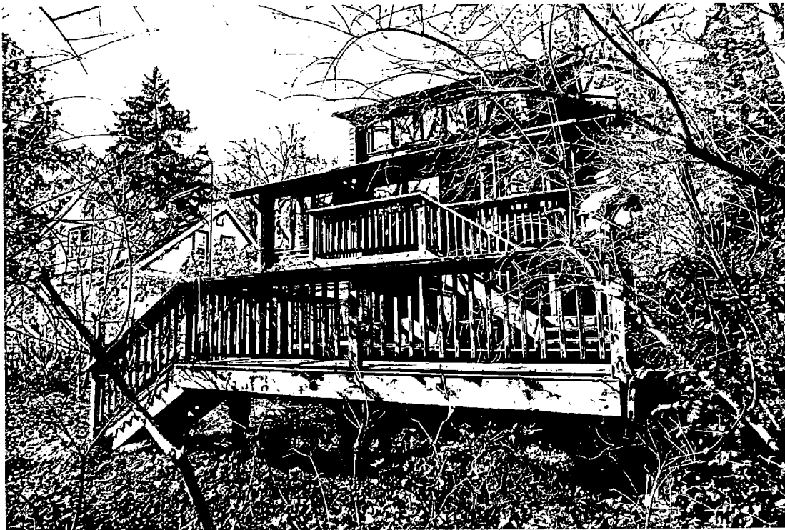
Detail: Rear view of the house right side of the deck from the backyard. The existing top deck to be converted into a screen porch.
