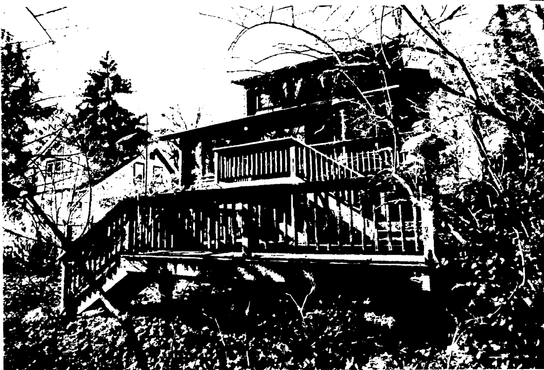
Detail: rear view of the house right side of the deck from the backyard. the existing top deck to be converted into a screen porch.
