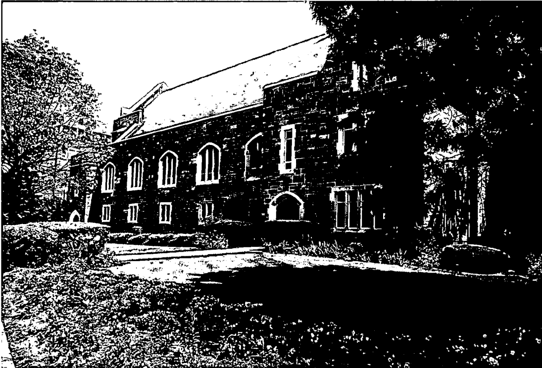
6951 Carroll Avenue, side (north) facade.
