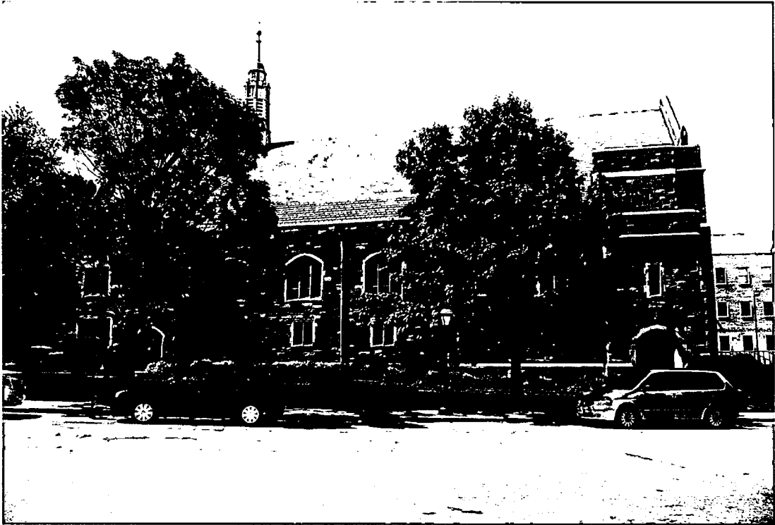
6951 Carroll Avenue, Side (north) Facade
