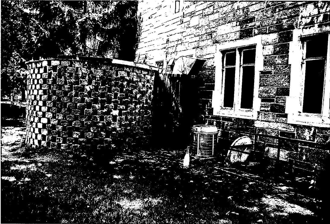
6951 Carroll Avenue, Stone Enclosure - current Conditions.
