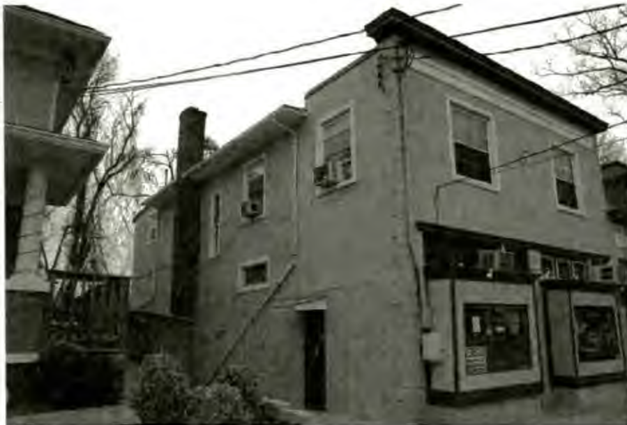
7040 CARROLL AVE EXISTING FRONT/LEFT FAÇADE
