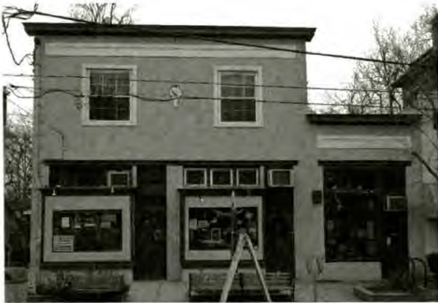
7040 CARROLL AVE EXISTING FRONT FAÇADE
