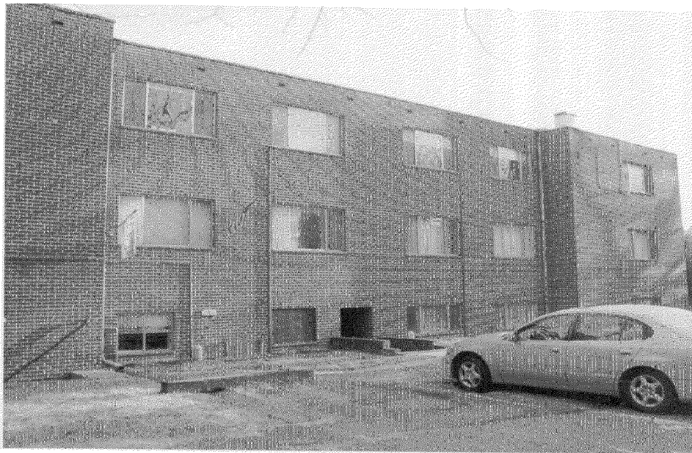
Rear View of Building – 407 Tulip Avenue
