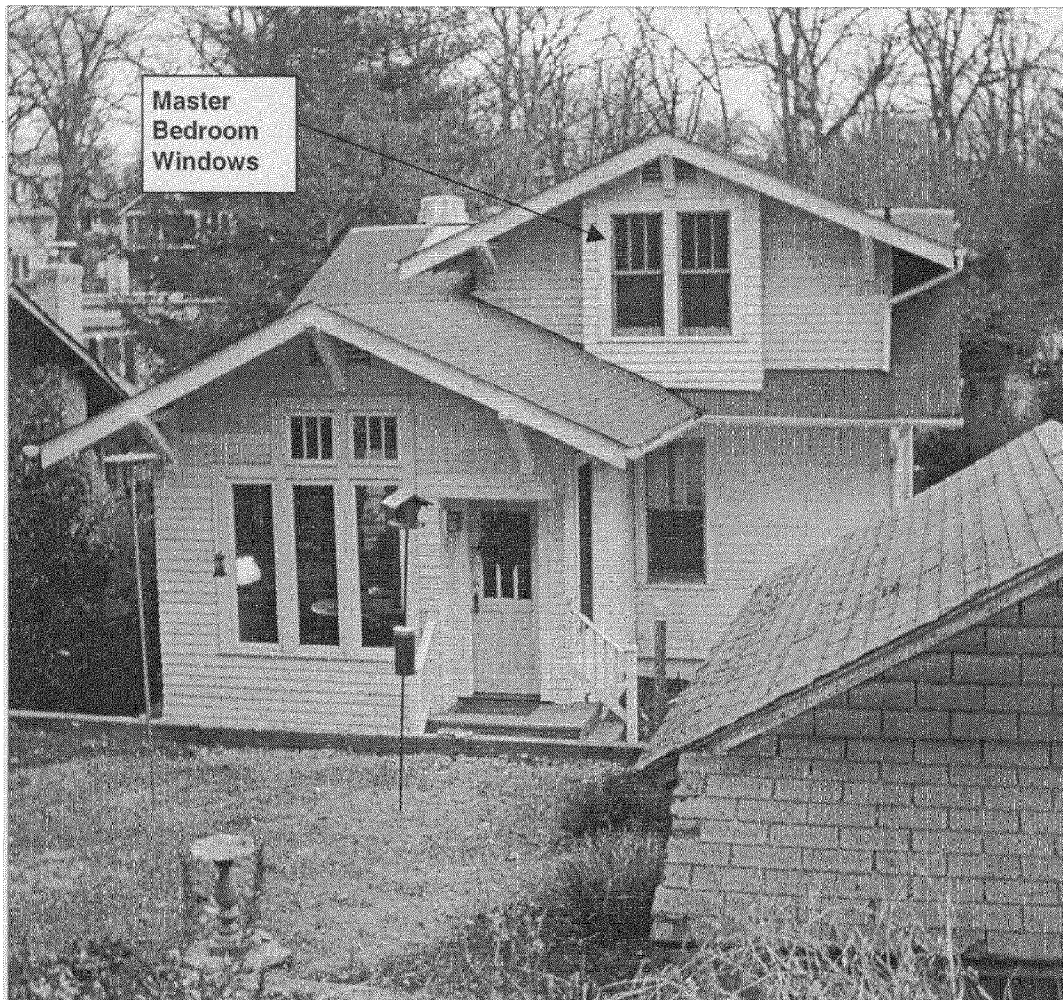
Rear Elevation View 7312 Willow Avenue Takoma Park View from A on Project 1 Site Plan
