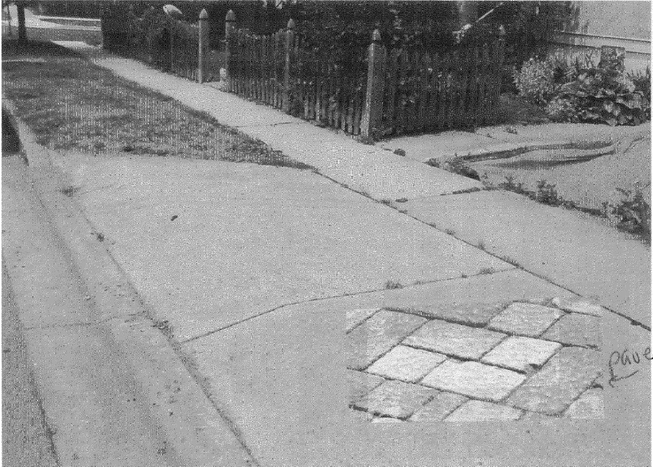
existing apron on street
