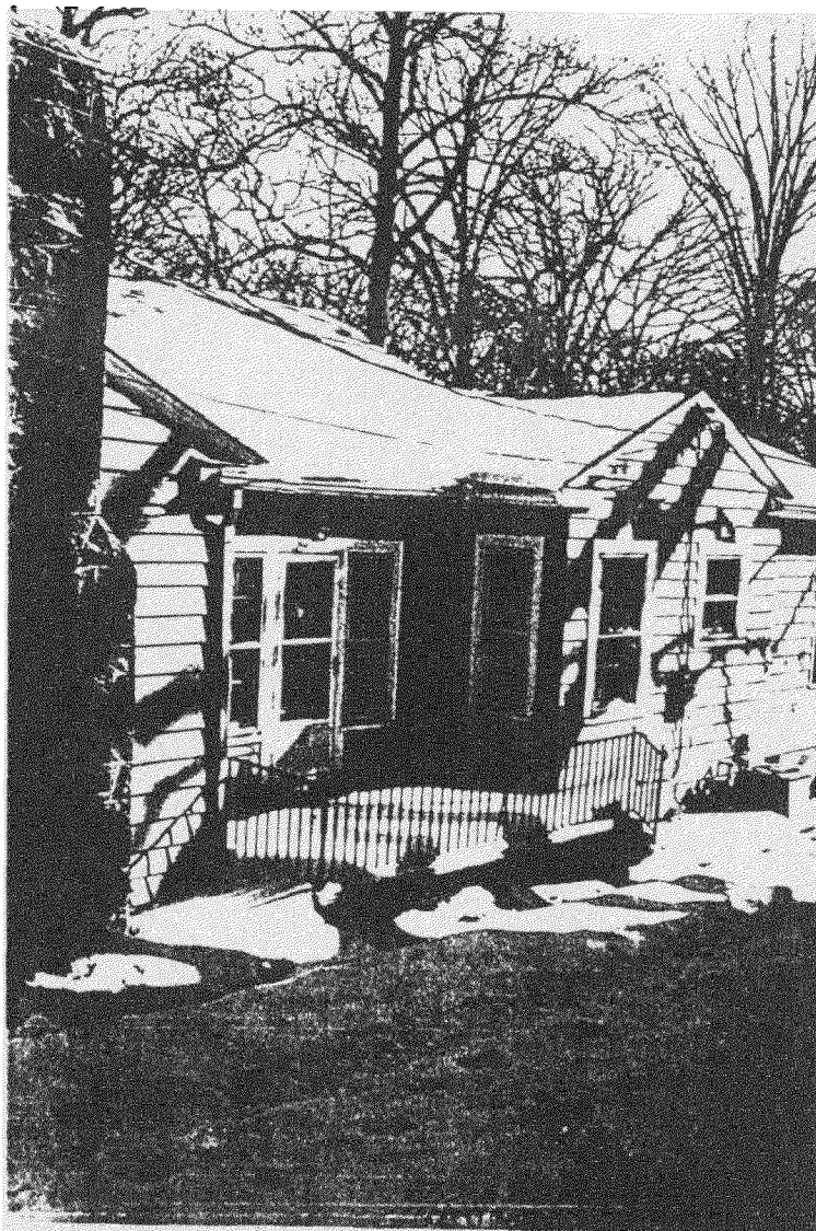
VIEW OF EXISTING CONCRETE PATIO TO BE ENCLOSED FROM 7209 WILLOW
