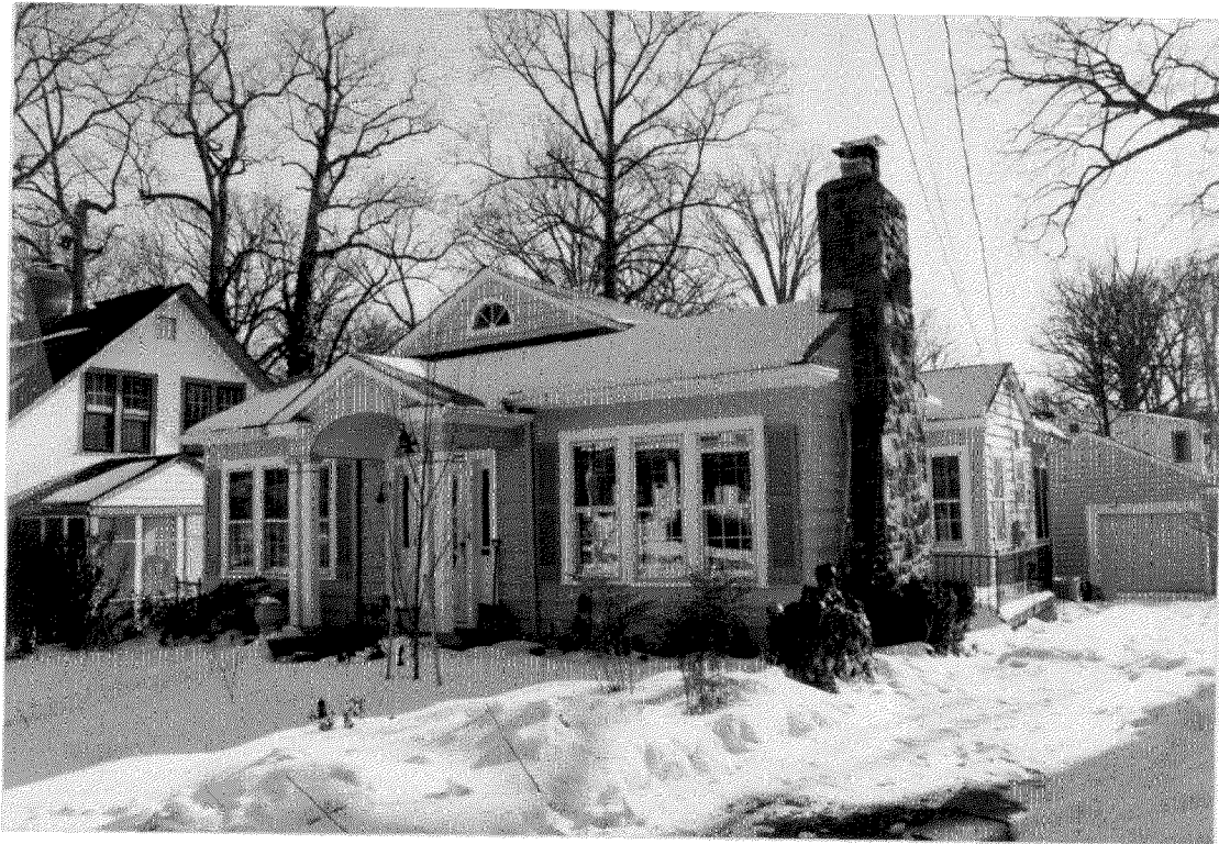
VIEW OF 7211 WILLOW, SCREENED PORCH OF 7213 WILLOW & PARTIAL VIEW OF EXISTING CONCRETE PATIO
