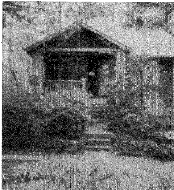
7314 WILLOW AVE FRONT FACADE
