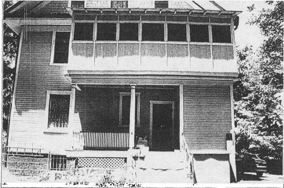
Rear portion of the existing house as seen from the back yard.
