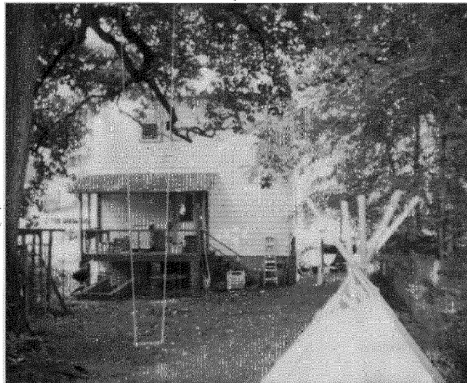
VIEW OF REAR
