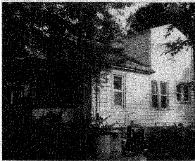
(SOUTHEAST) SIDE VIEW
